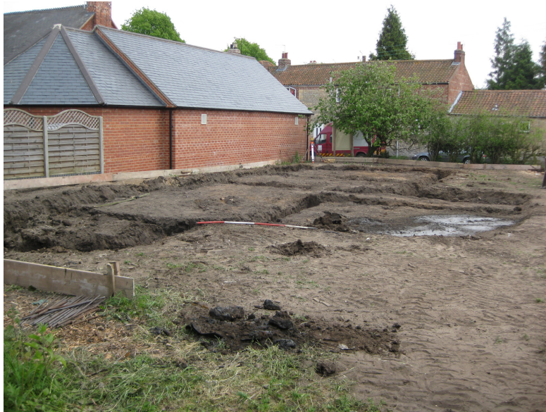
Plate 1 – General view across the development area, looking southeast
