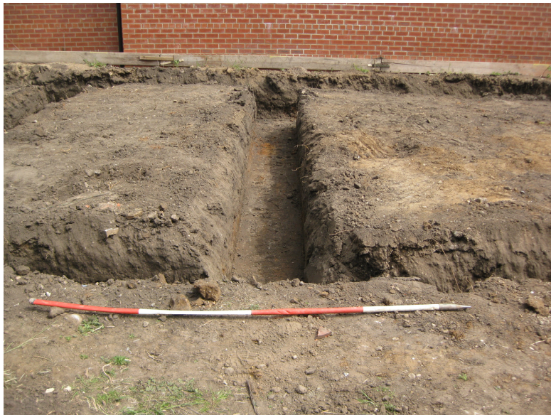
Plate 2 – Detail of foundation trenches showing the general sequence of deposits, looking east
