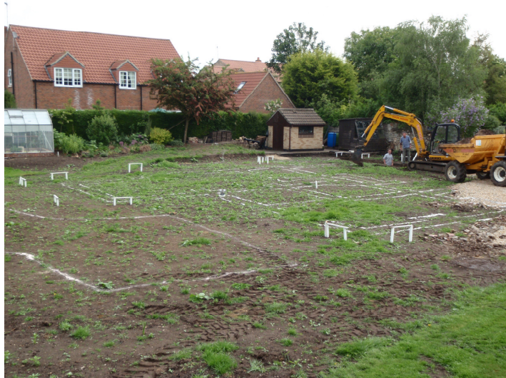
Plate 1 – General view across the site, looking northeast
