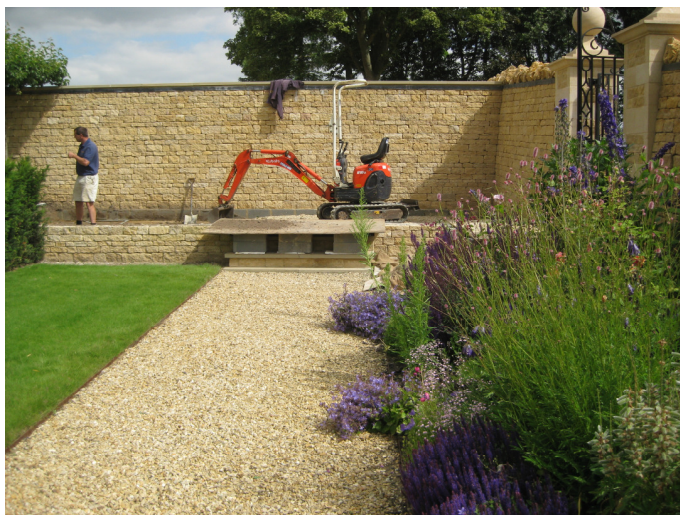
Plate 4 – View looking north towards the summerhouse area
