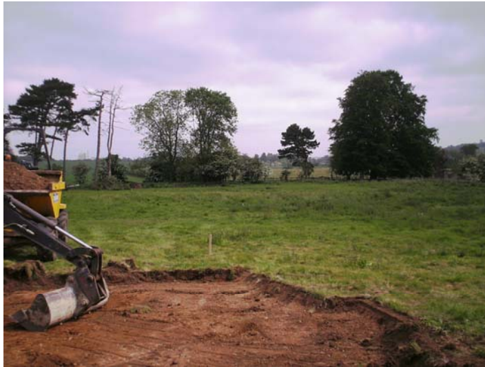
Plate 1 – General view across the area of works, looking northwest
