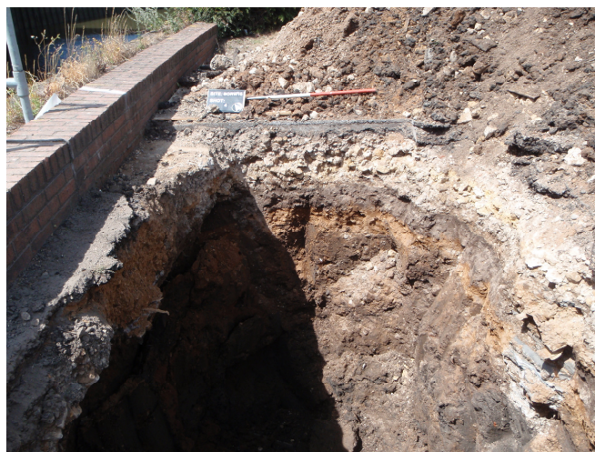
Plate 3 – Section 1, looking north
