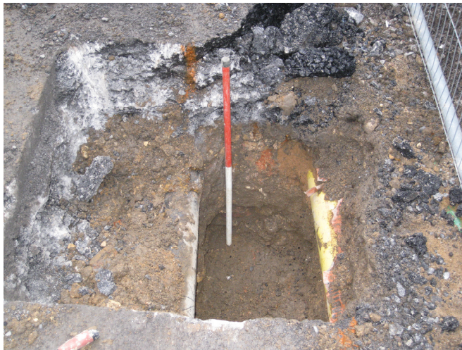
Plate 2 – Section 2, looking south
