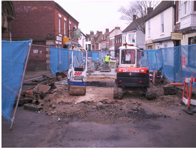
Plate 1 – View looking north along Bailgate
