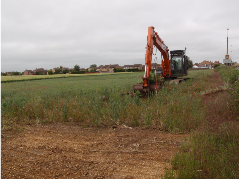
Plate 1 General site view, commencement of machine stripping, looking west
