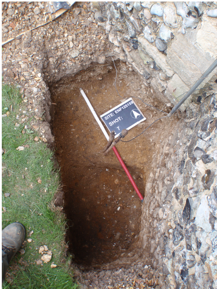
Plate 2 – Trench 1 after excavation, looking north
