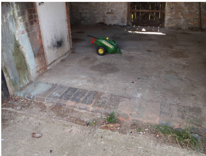
Plate 23 Detail of flooring inside barn, ceramic tiles at threshold and concrete beyond, looking south
