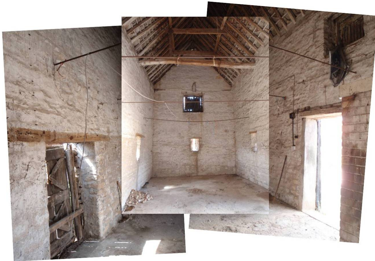
Plate 14 Interior of barn, looking west
