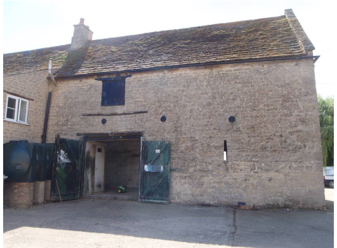
Plate 11 North elevation of barn, looking south
