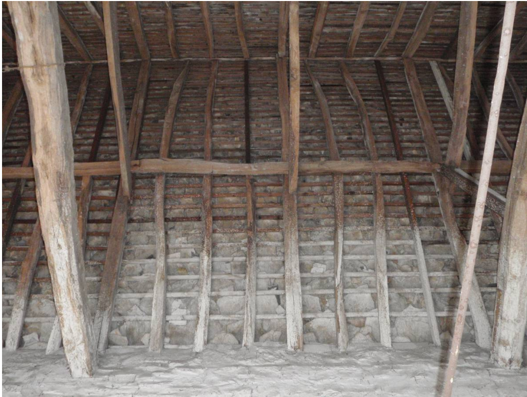
Plate 16 Interior of barn showing detail of roof construction, looking south
