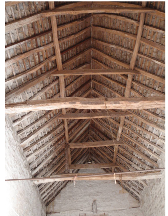
Plate 15 Interior of barn showing roof construction, looking west
