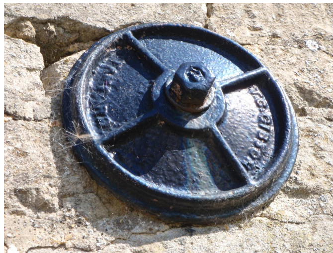
Plate 8 Detail of south elevation of barn showing breather slit, roofing and cross tie plate, looking north
