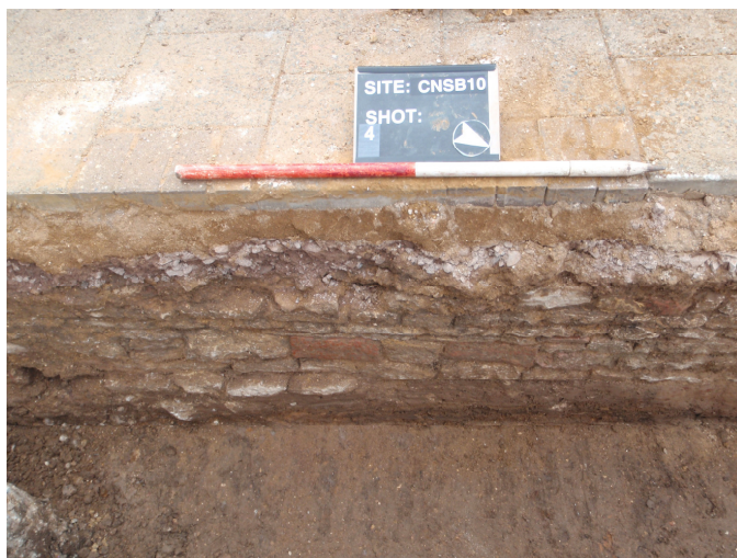
Plate 3 – Section 1 with wall (005), looking southwest
