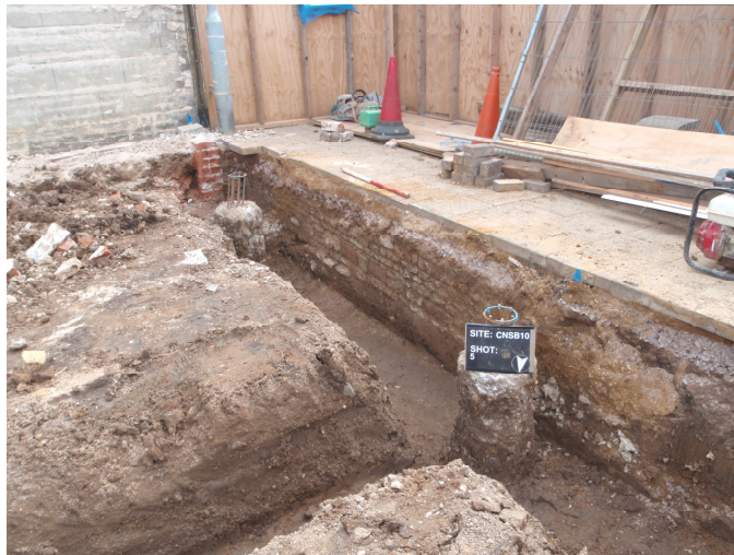
Plate 2 – Wall (005), looking south
