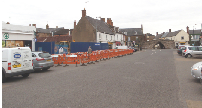
Plate 1 – View showing the development area with Trinity Bridge in the background, looking southeast
