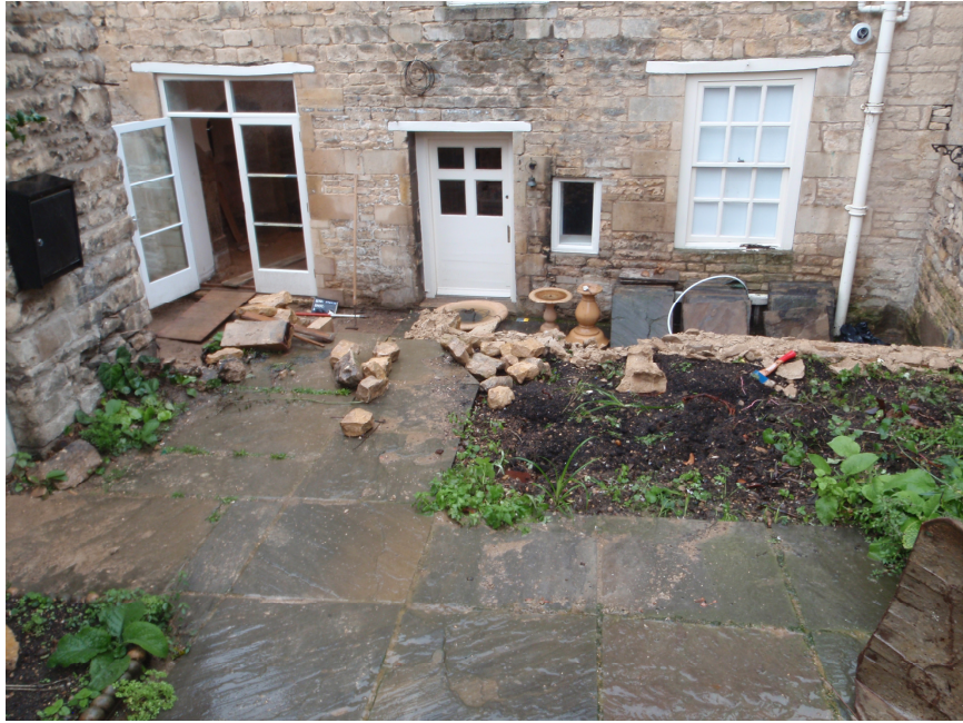
Plate 1 – General view of the development area prior to works, looking northeast
