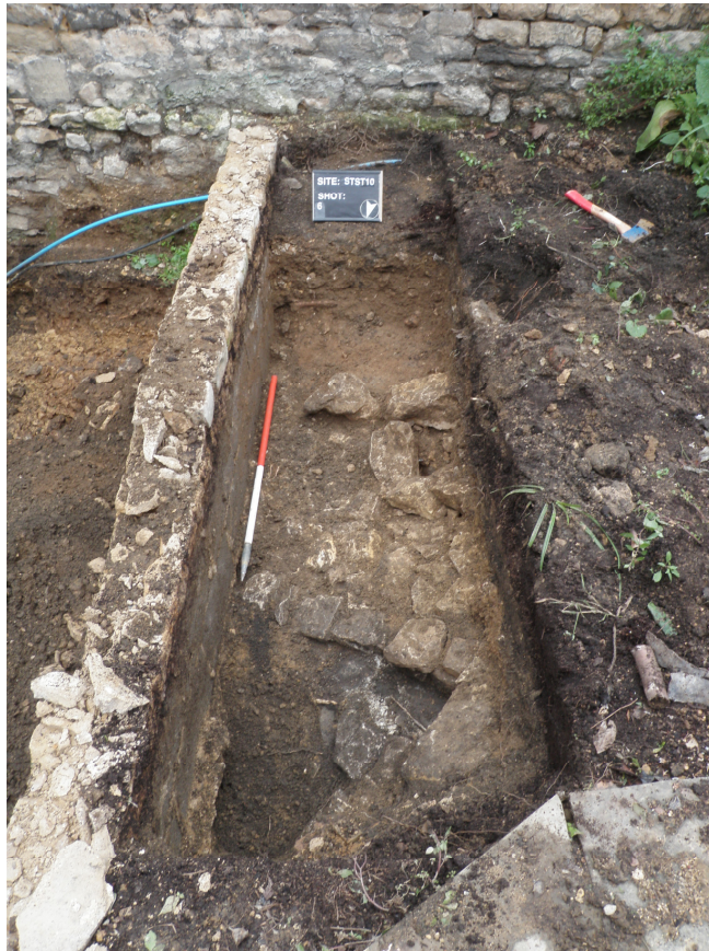
Plate 3 – View after the removal of overburden showing the stone drain (012), looking southeast
