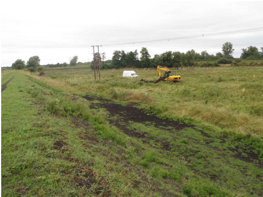
Plate 2. Machining Trench 8 looking north from Reach Lode bank towards Burwell Lode
