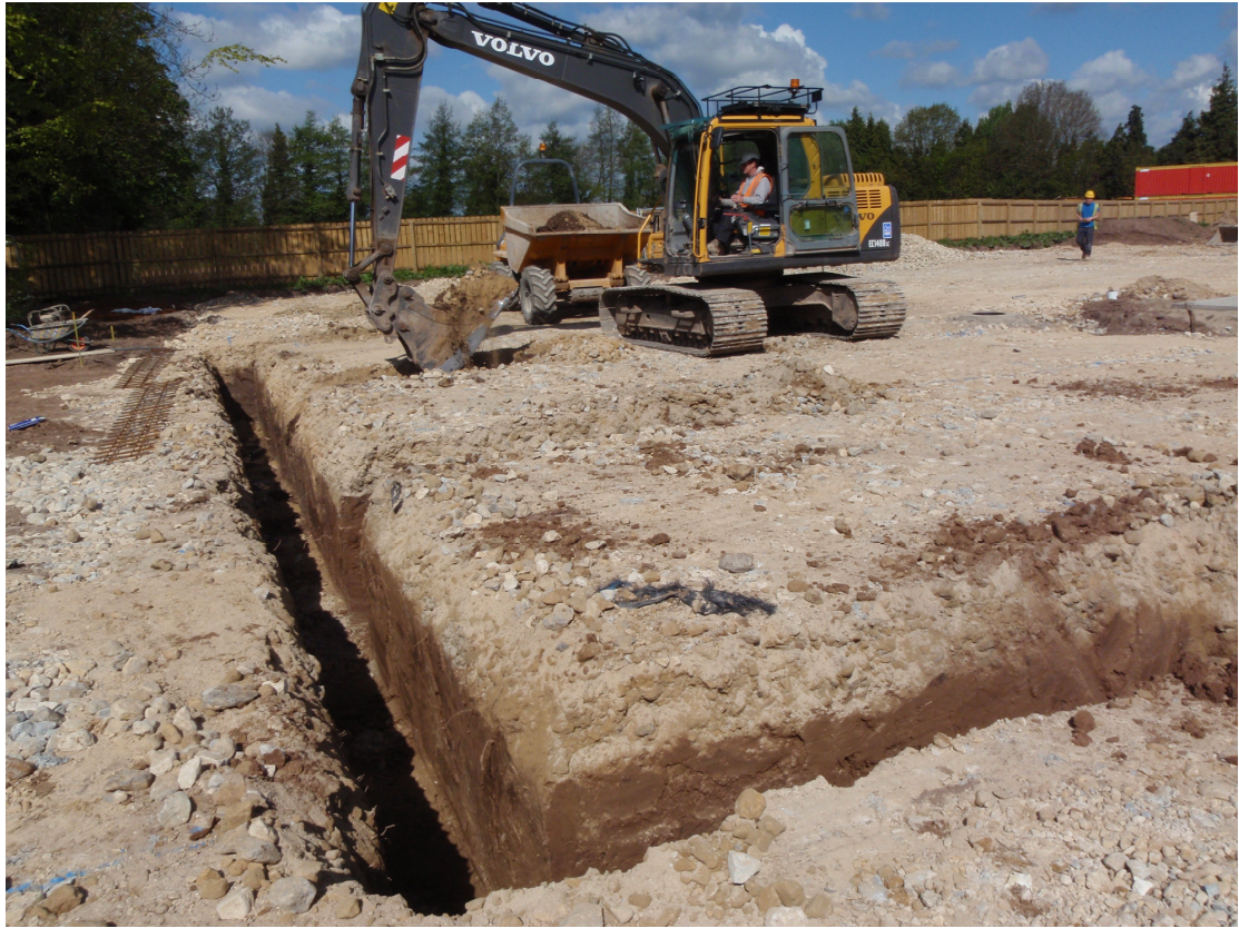
Plate 5. Machining of footings of Plots 18-20 looking west
