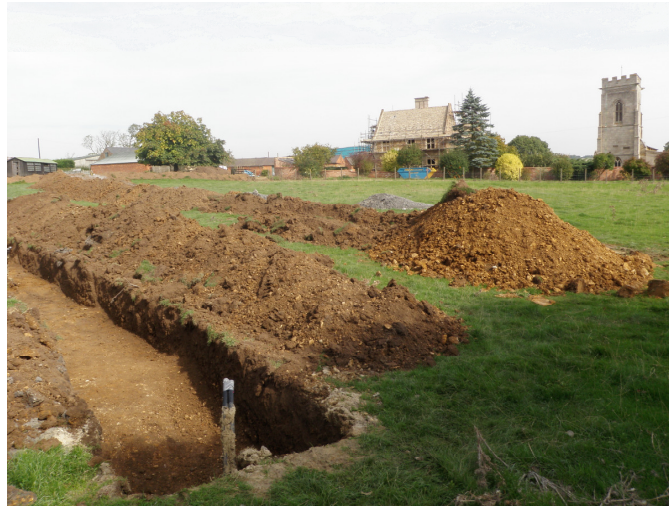
Plate 1 – General view across the site towards the Old Hall and St Peter's church, looking northeast
