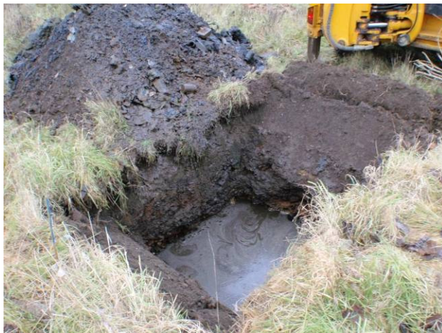
Plate 3 Trench 1, showing build up of dumped material.
