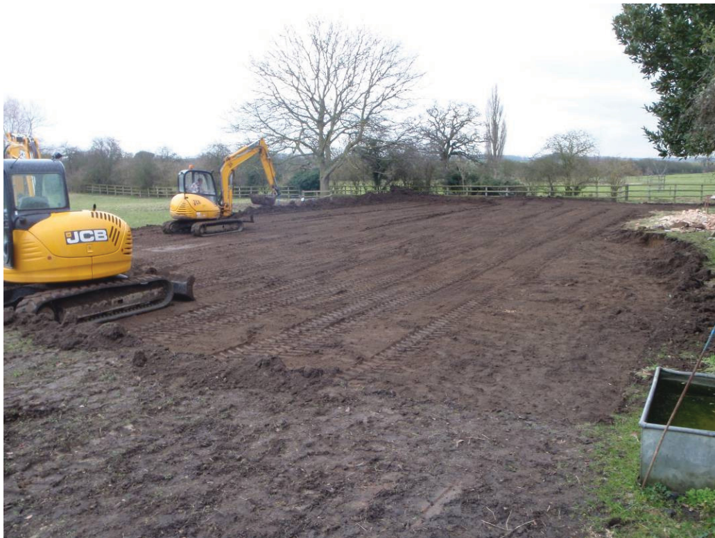
Plate 4 Site on completion of earthmoving
