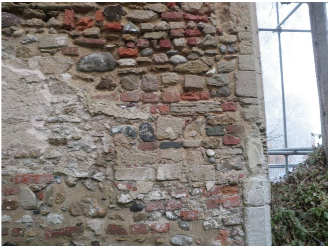
Plate 14. St Peter's observation Point 5 on north side of nave
