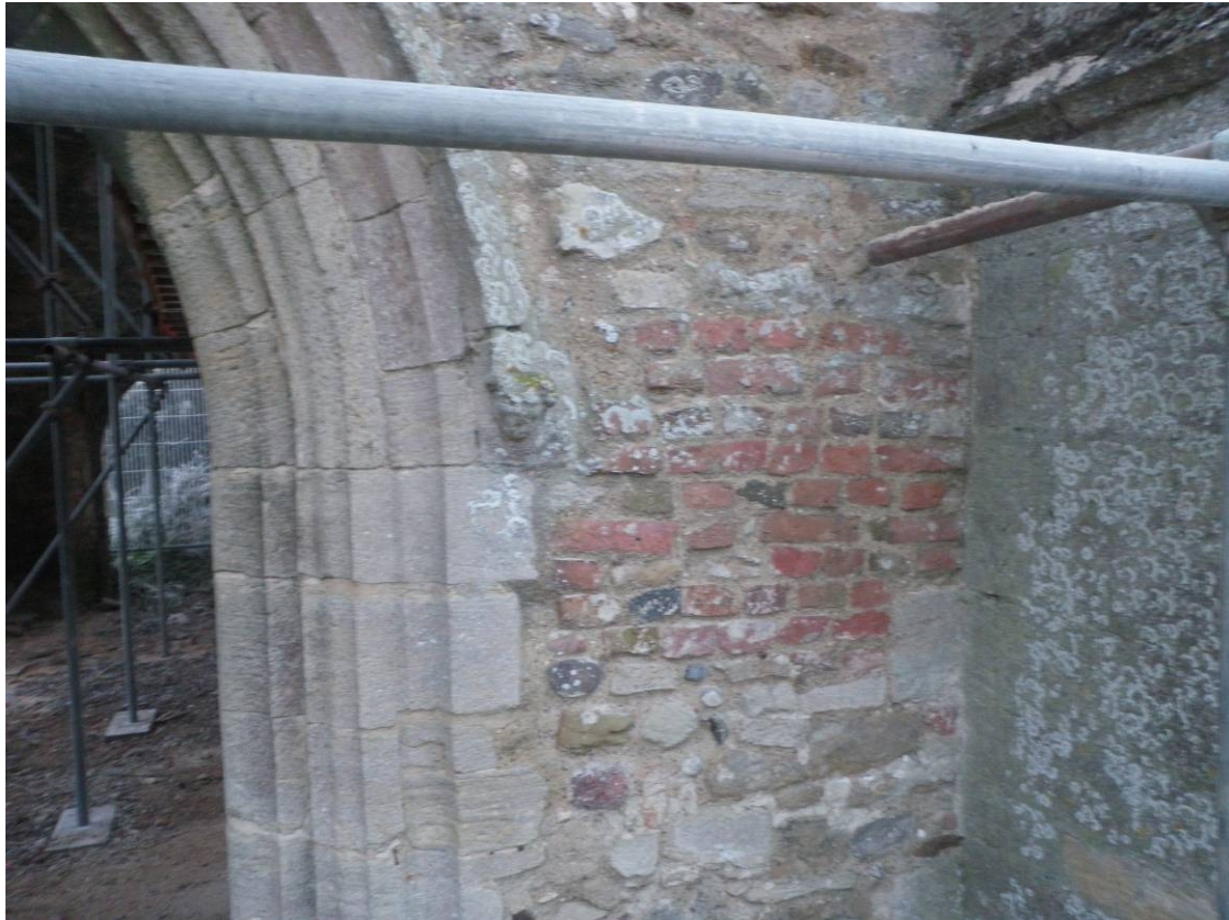
Plate 15. St Peter's observation Point 6 on north side of tower
