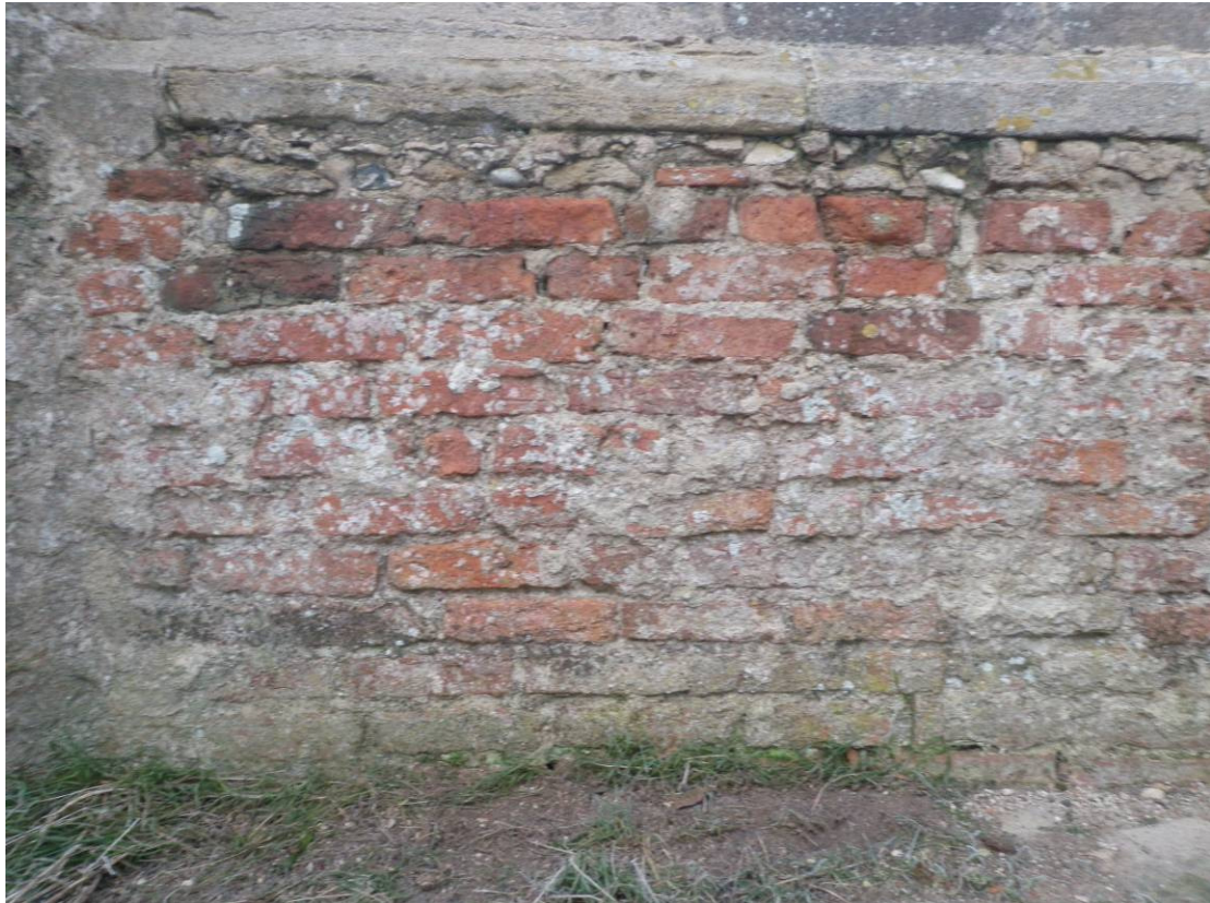
Plate 13. St Peter's observation Point 4 on north side of nave
