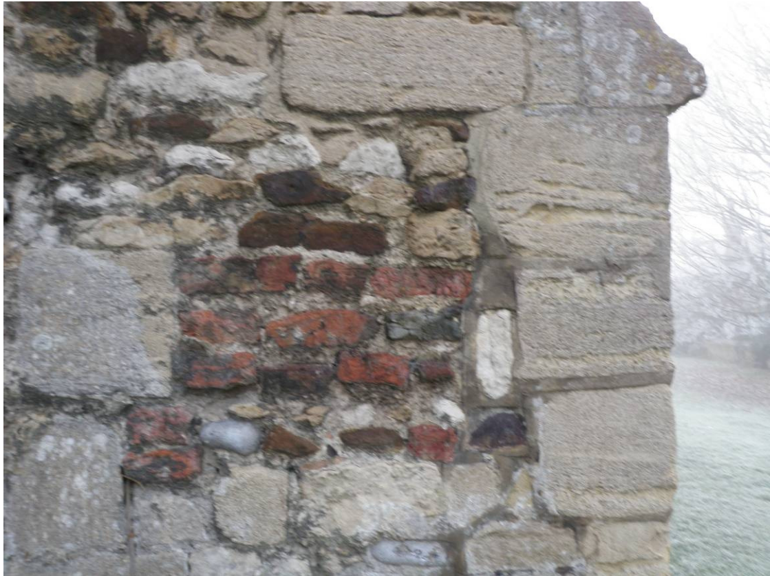
Plate 3. St Mary's observation Point 2, buttress of west tower
