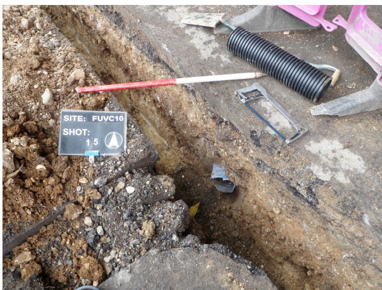
Plate 3 – Section 4, looking southeast
