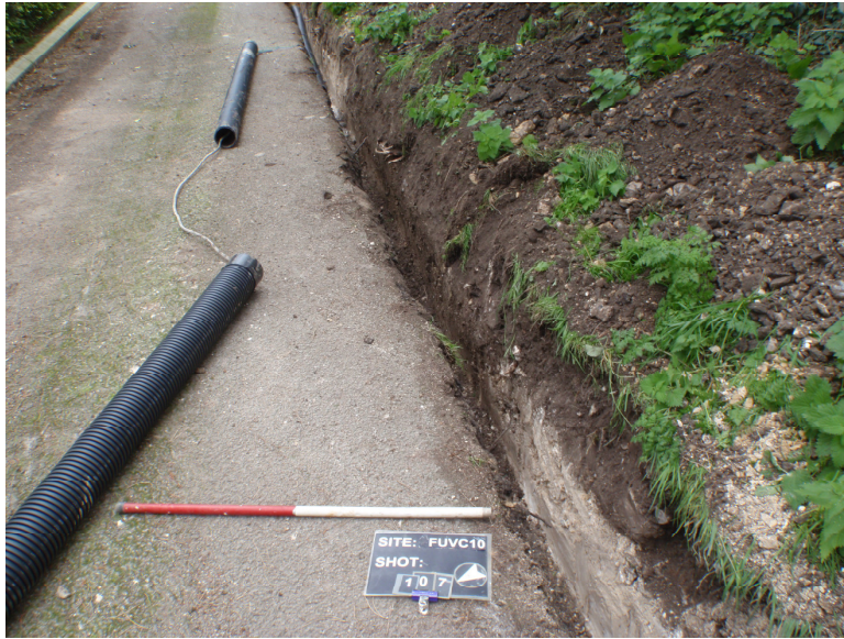
Plate 7 – Section 41, looking southeast
