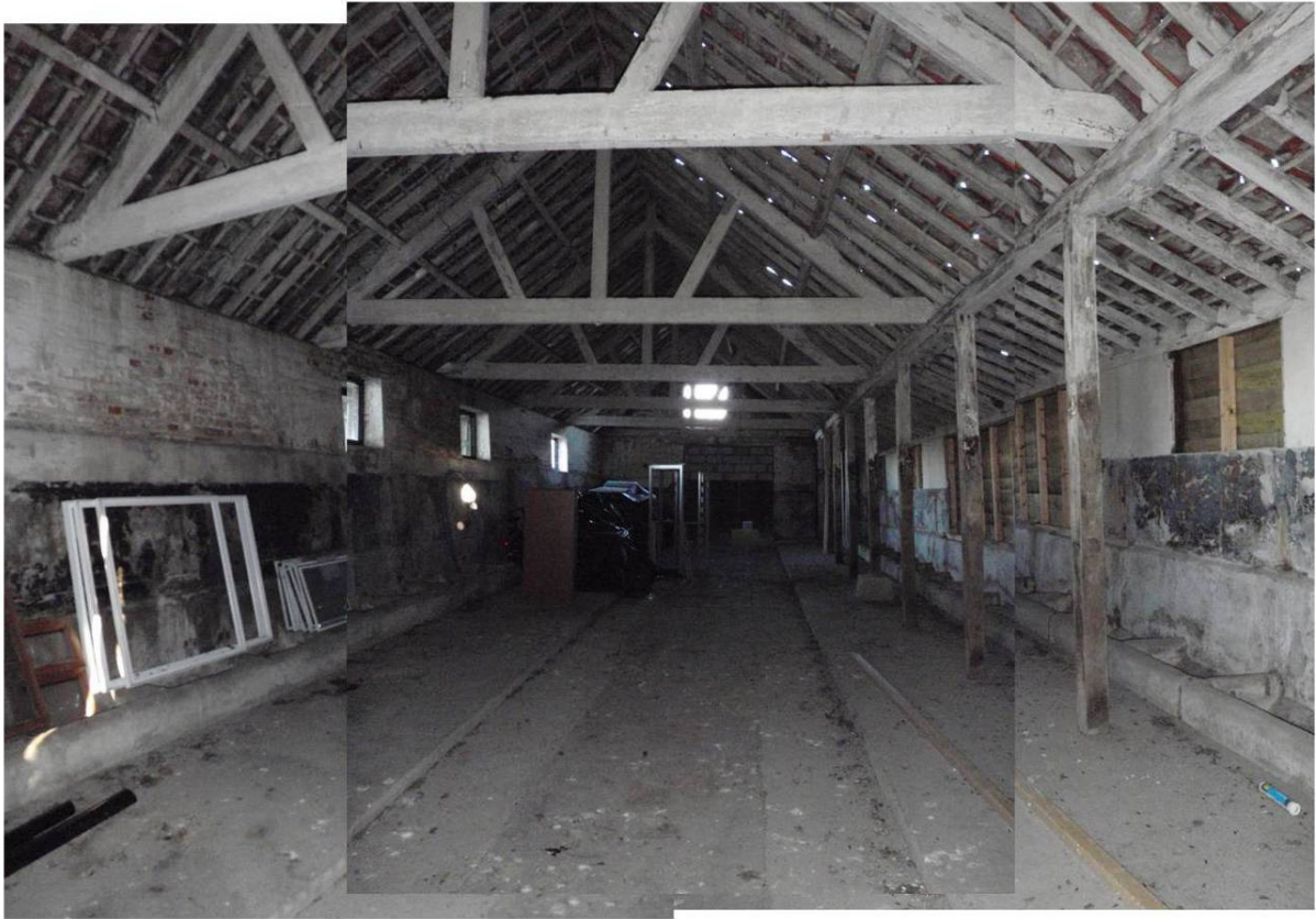
Plate 38 Interior of main room, Range 1, general view, looking northeast
