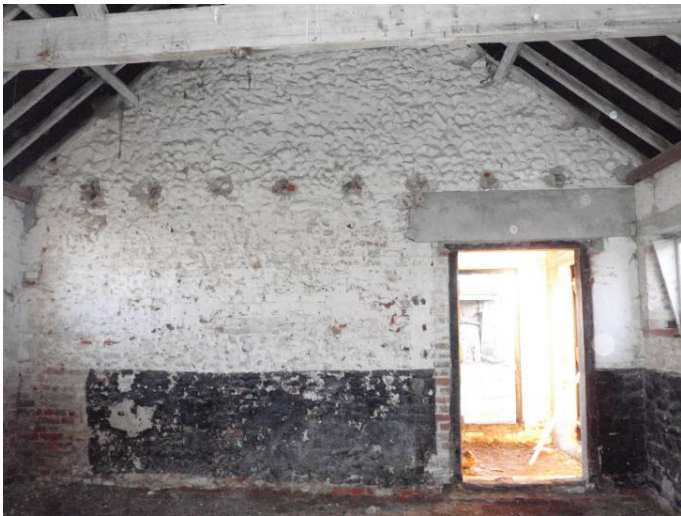
Plate 28 Interior of Range 2, central room, wall 2e, showing joist holes, looking southwest
