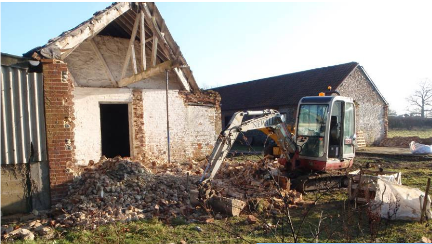
Plate 41 General view showing partial demolition of Range 1 in progress, looking southeast
