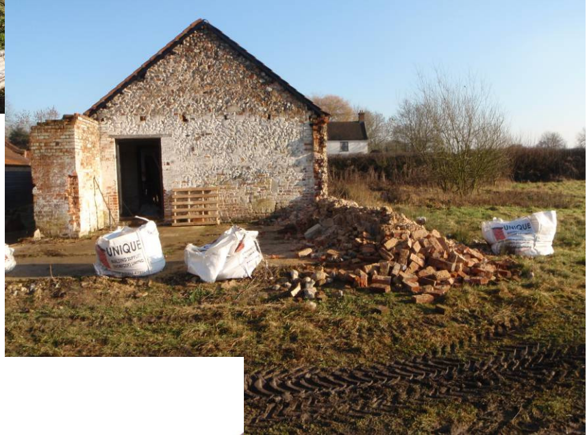
Plate 42 General view showing Range 2, partially demolished, looking northeast
