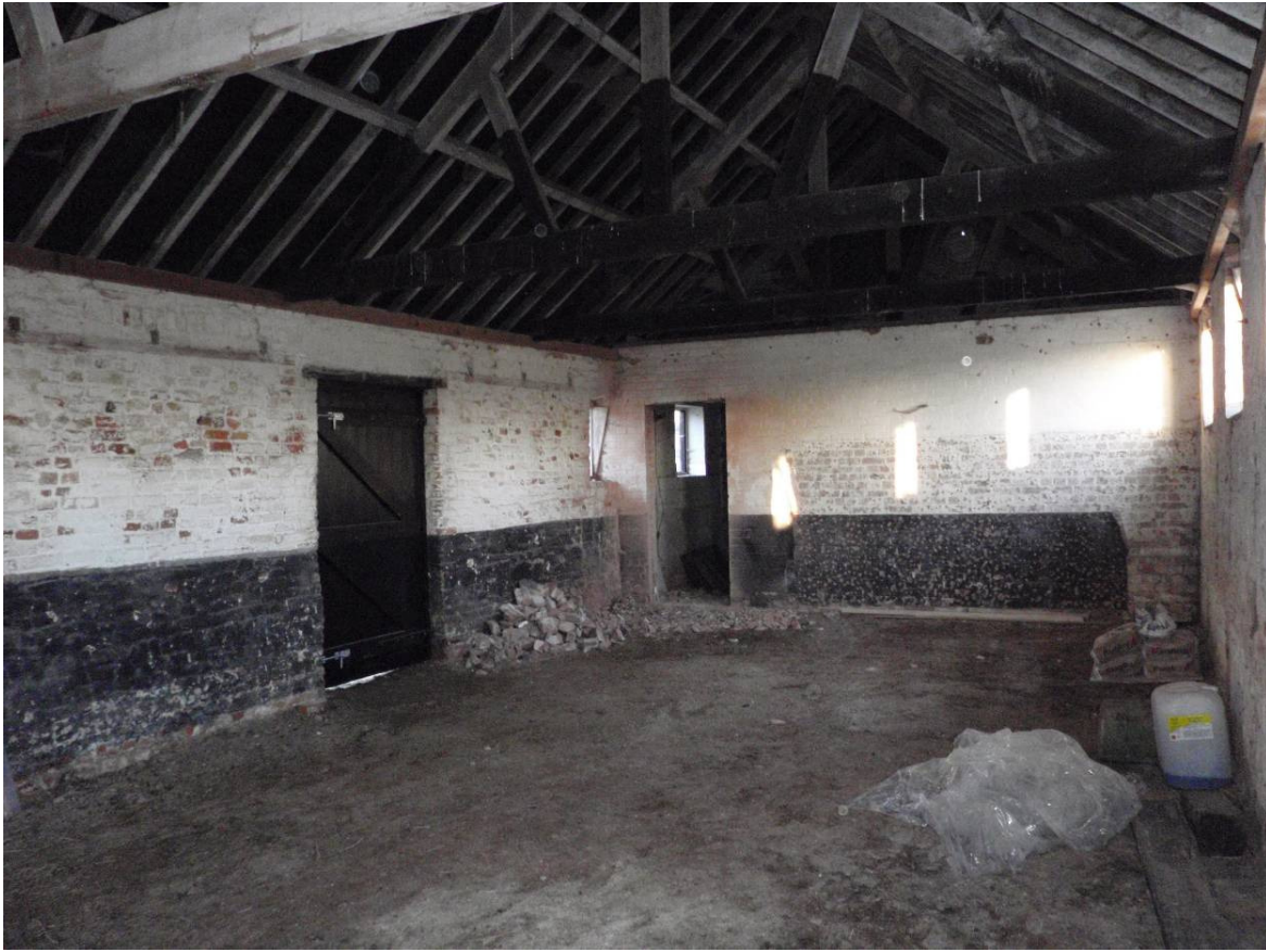
Plate 27 Interior of Range 2, central room, walls 2a and 2f, looking northeast
