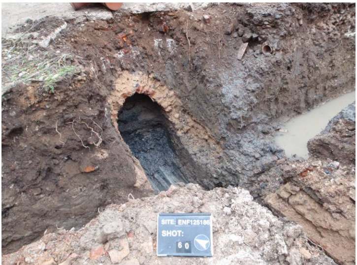
Plate 48 Brick culvert 041, drain within [040] visible at top right, looking south
