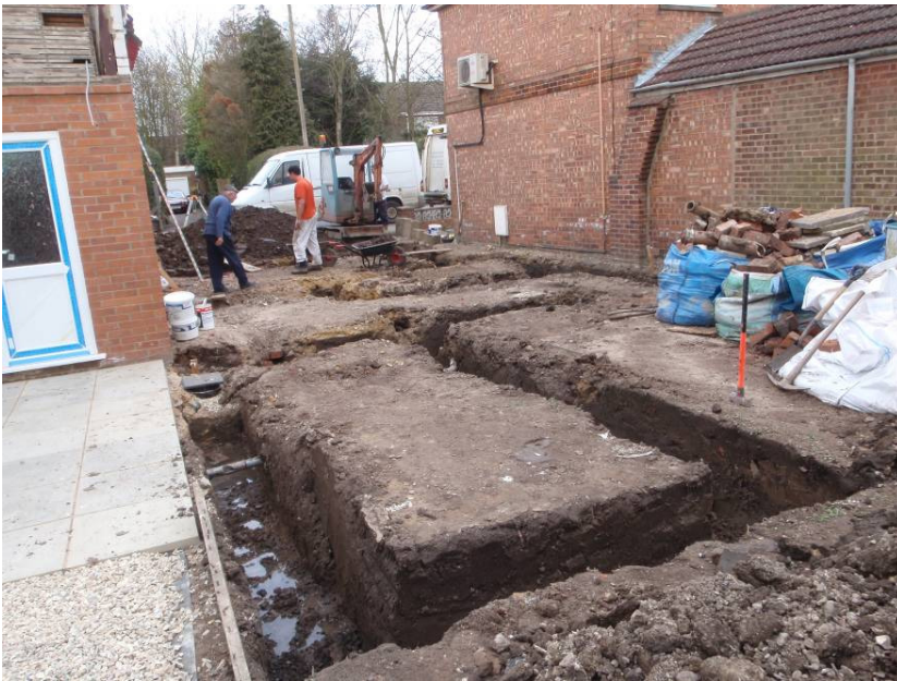
Plate 2 General view of site, looking northeast
