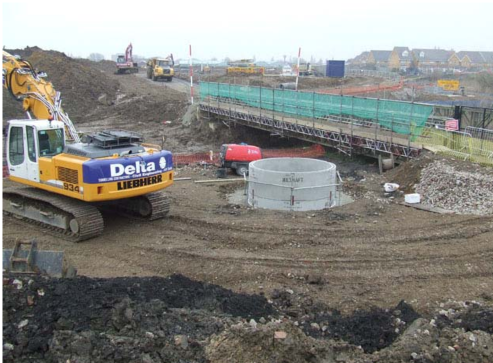
Plate 2: Washout chamber shaft
