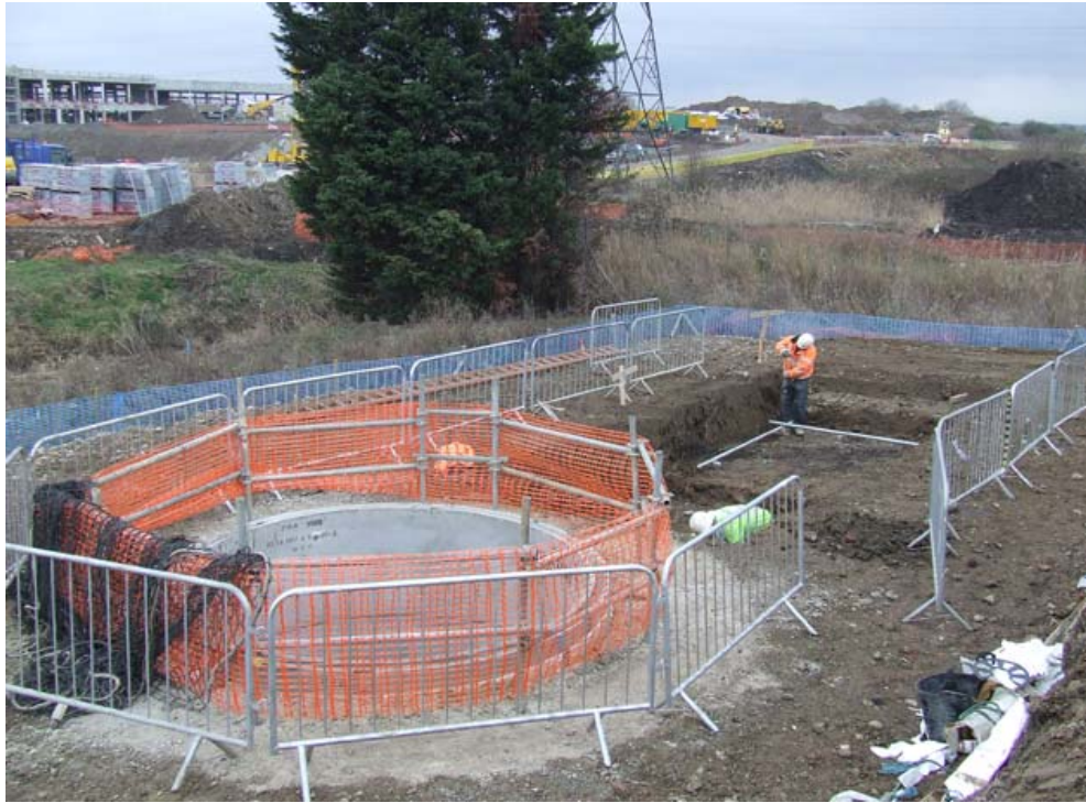
Plate 1: Pump station shaft
