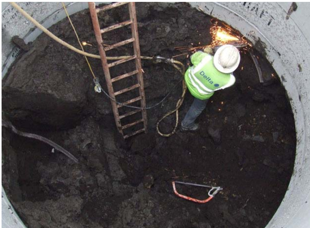
Plate 4: Peat at washout chamber shaft
