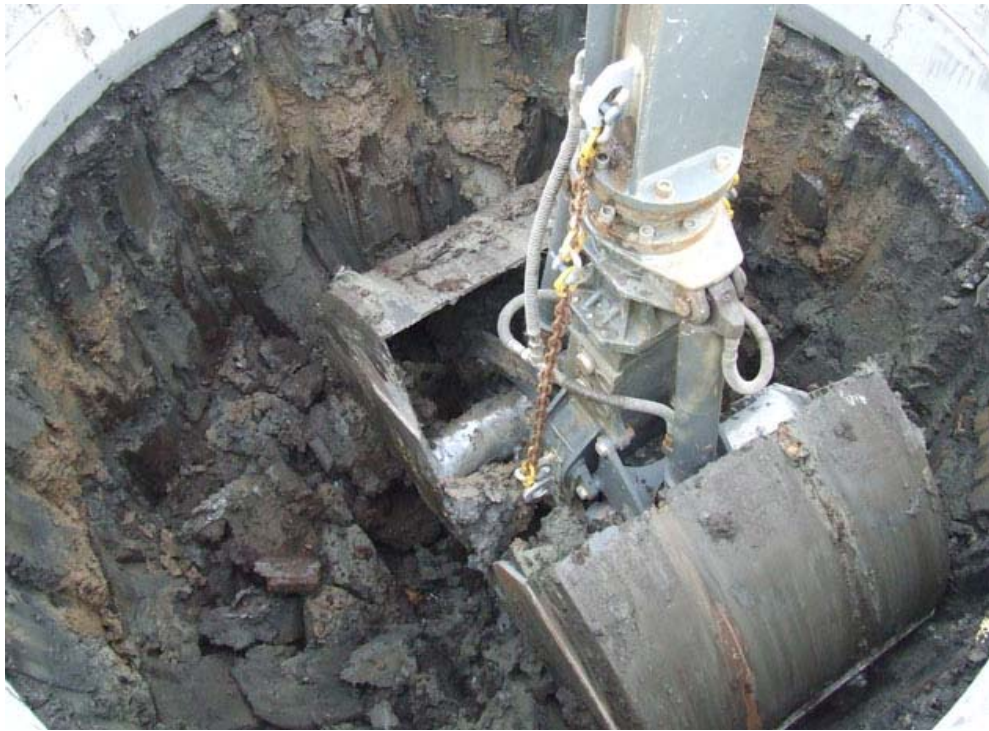
Plate 3: Mechanical excavation of lower alluvium at pump station shaft
