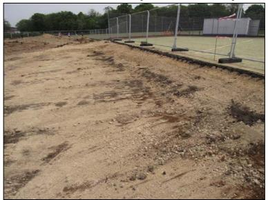
Plate 2: Made ground under the existing all weather pitch
