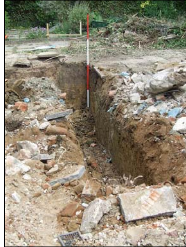
Plate 1: General shot of southern footing trench, looking east, 2m scale
