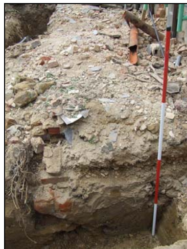
Plate 3: Wall footing in east footing trench, looking west, 2m scale
