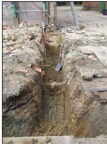
Plate 2: Eastern footing trench, showing cast iron pipe, 2m scale
