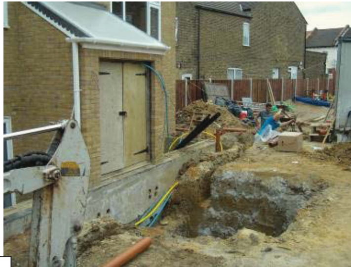
Plate 3: southern drain trench and waste tank pit
