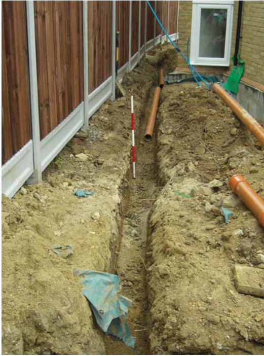
Plate 1: Western drain trench
