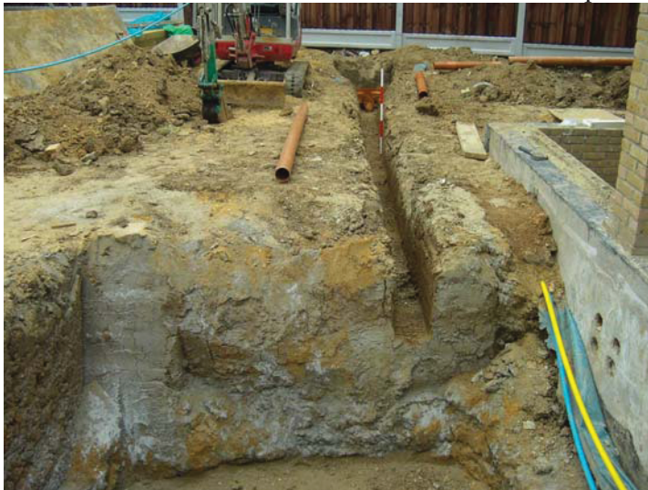
Plate 4: Southern drain trench and waste tank pit
