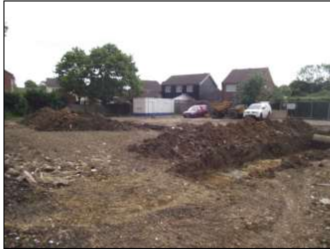
Plate 1: General view of the site during the fieldwork
