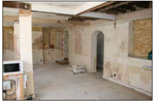
Plate 14: Room G3: south wall
