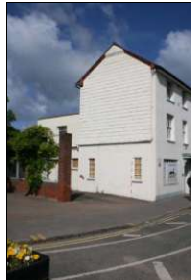
Plate 4: East elevation of main building
