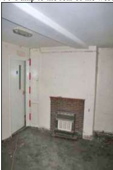
Plate 11: Room G2: southwest corner
