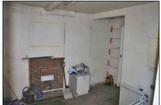
Plate 10: Room G1: northwest corner
