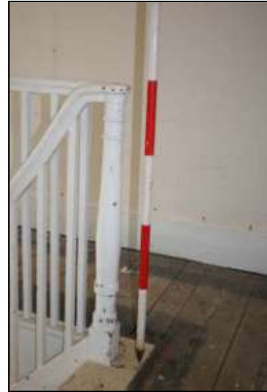
Plate 32: Room S1: stair detail
