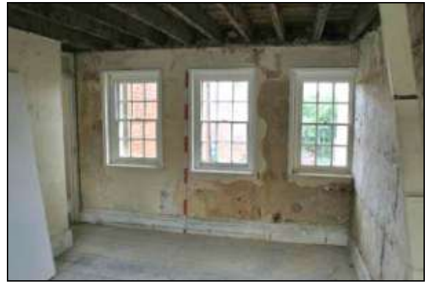
Plate 26: Room F5: south wall
