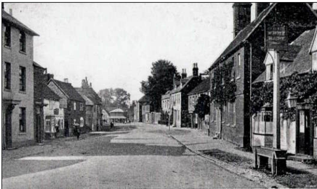
Figure 7: Photograph of the High Street in 1899 (from McFarlane 1984)
