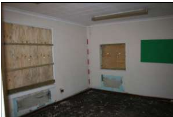
Plate 17: Room G4: southeast corner
