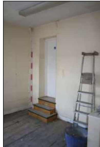
Plate 28: Room F6: northeast corner
