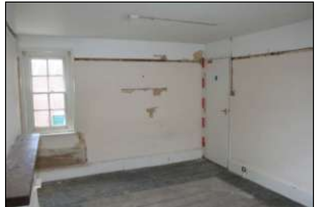
Plate 22: Room F3: looking southwest
