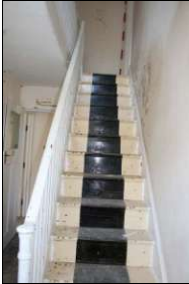
Plate 19: Room F1: staircase to second floor
