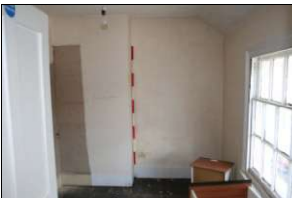
Plate 35: Room S3: southwest corner
