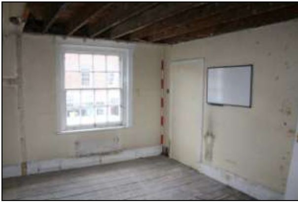
Plate 25: Room F5: northeast corner
