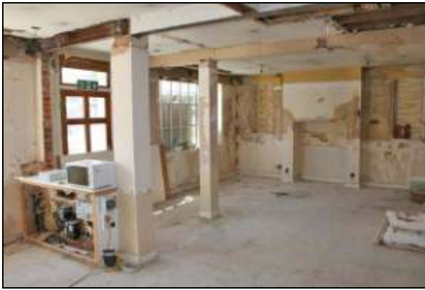
Plate 13: Room G3: north wall
