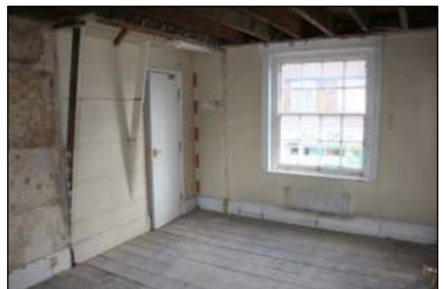
Plate 24: Room F5: northwest corner
