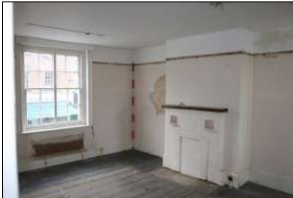
Plate 21: Room F3: northeast corner
