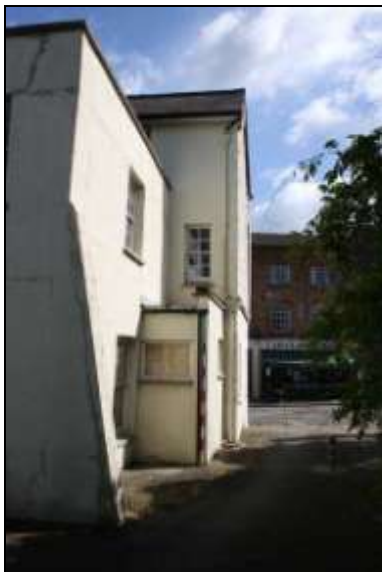
Plate 5: East elevation of rear extension
