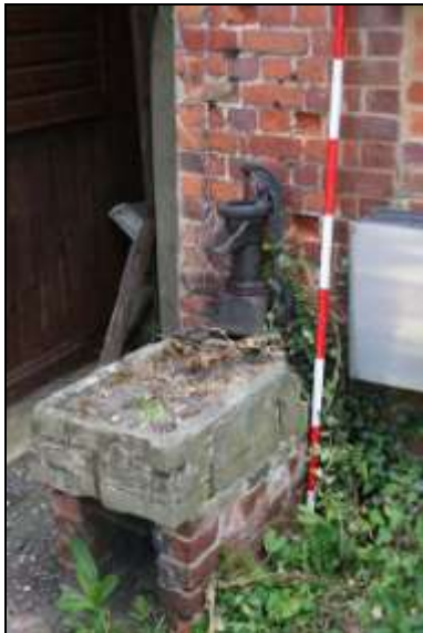
Plate 9: Pump to the rear of the west wing
