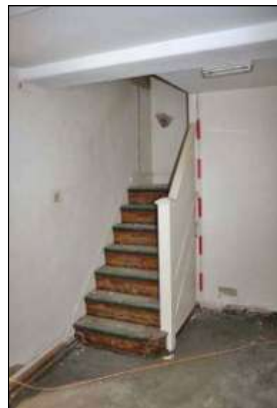
Plate 12: Room G2: southeast corner
