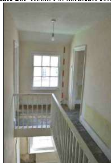
Plate 30: Room S1: north wall
