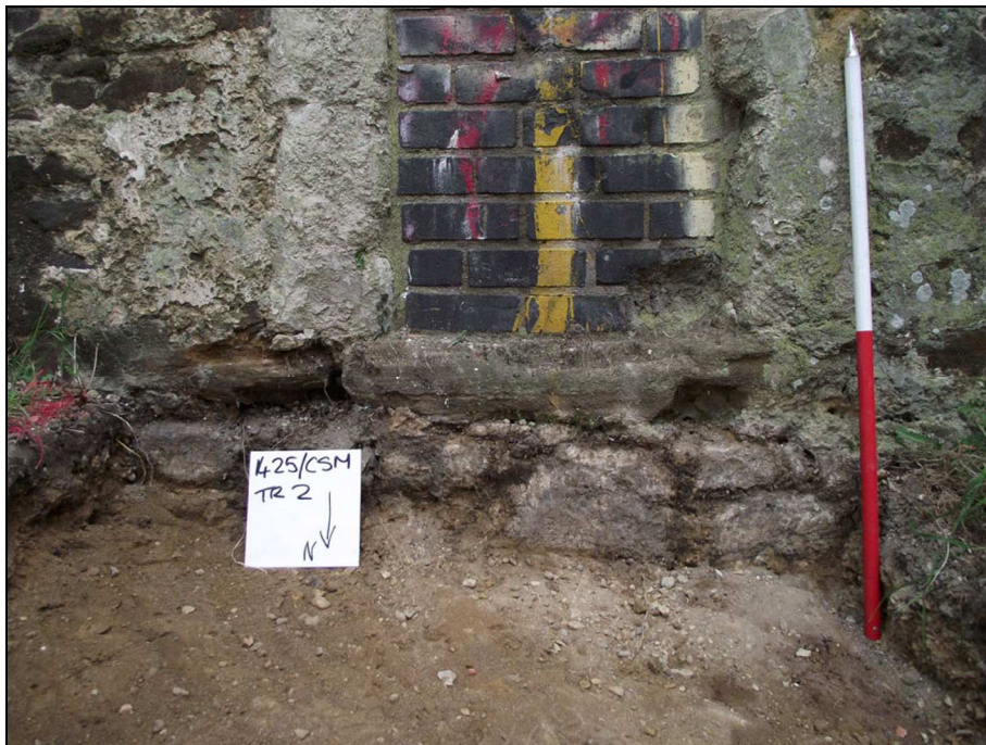
Plate 4: Trench 1: church foundations, looking S (scale 1m)
