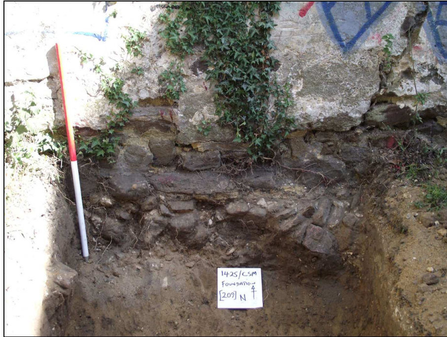
Plate 9: Trench 2: church foundations (209), looking N (scale 1m)
