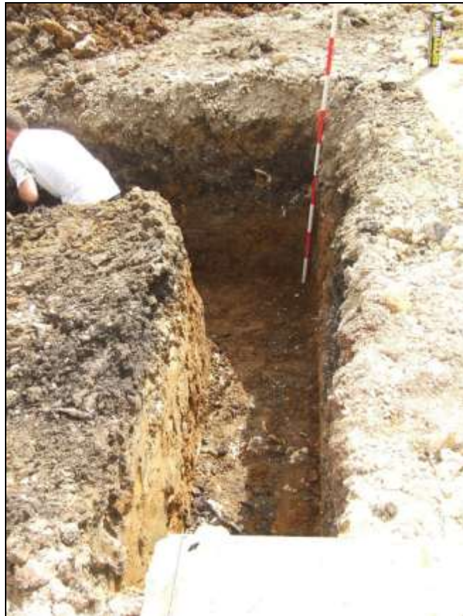
Plate 1: Footing trench, looking east, 2m scale
