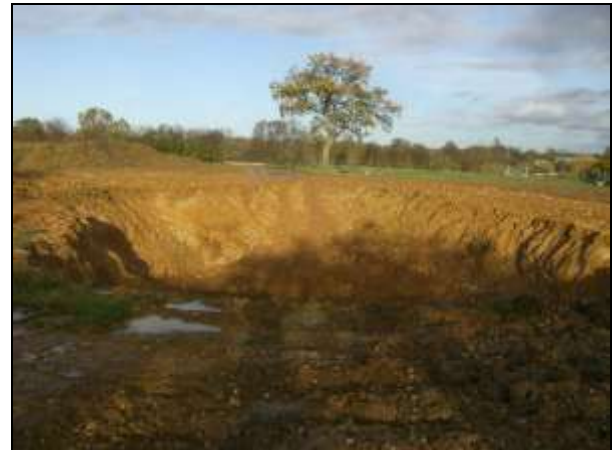
Plate 4: View NE across Pit G & H
