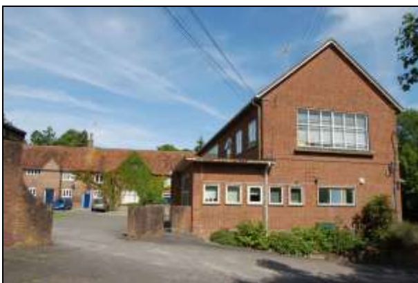
Plate 17: Buildings 4 & 6 from the south
