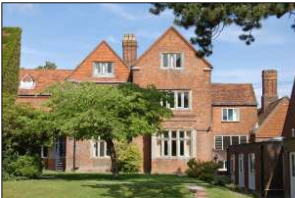
Plate 3: Building 1: south elevation
