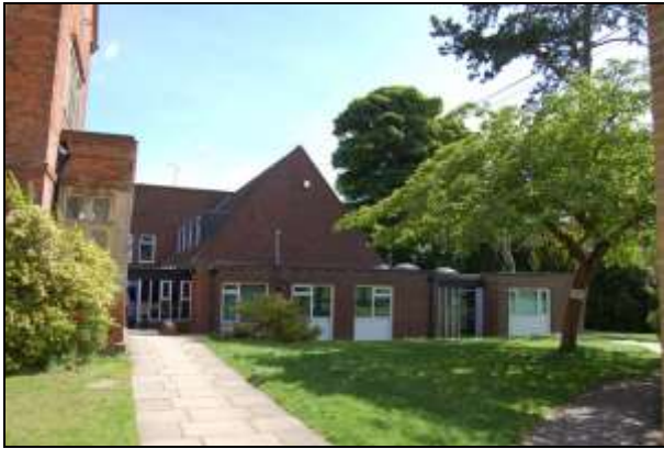
Plate 7: Building 2: west elevation
