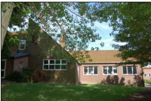
Plate 5: Building 2: south elevation
