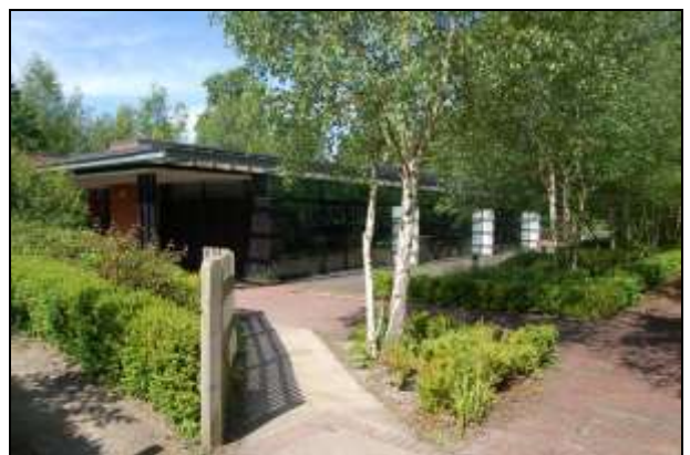
Plate 12: Building 5: view from the southeast
