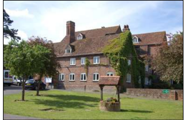
Plate 2: Building 1: east range
