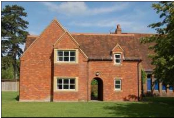
Plate 9: Building 3: south elevation
