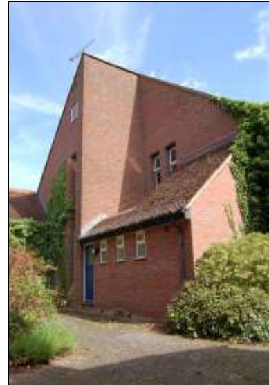
Plate 20: Building 7: west elevation
