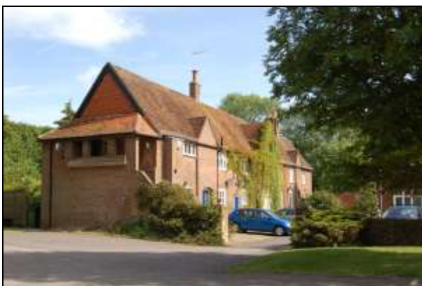
Plate 11: Building 4: west elevation
