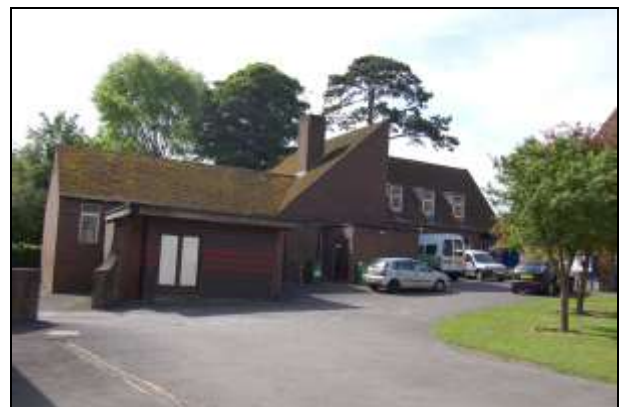
Plate 6: Building 2: north elevation
