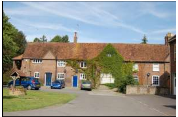
Plate 10: Building 4: south elevation
