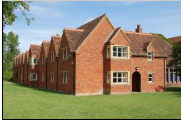
Plate 8: Building 3: view from the southwest
