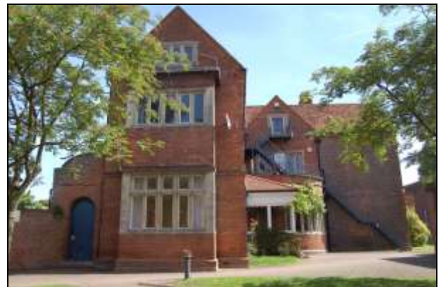
Plate 4: Building 1: west elevation
