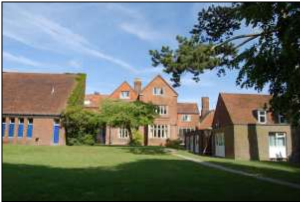
Plate 21: Buildings 1, 2 & 7 from the south
