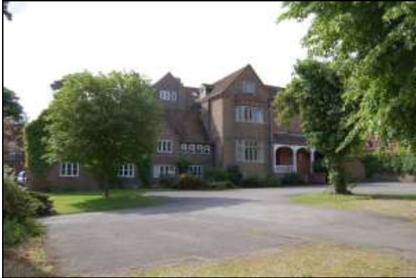
Plate 1: Building 1: north elevation
