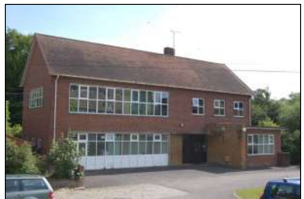
Plate 18: Building 6: west elevation
