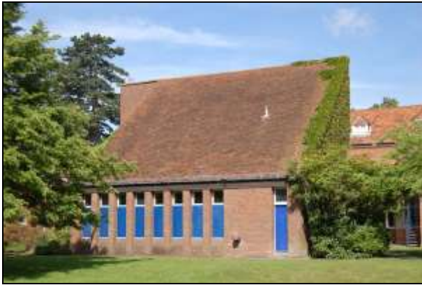
Plate 19: Building 7: south elevation
