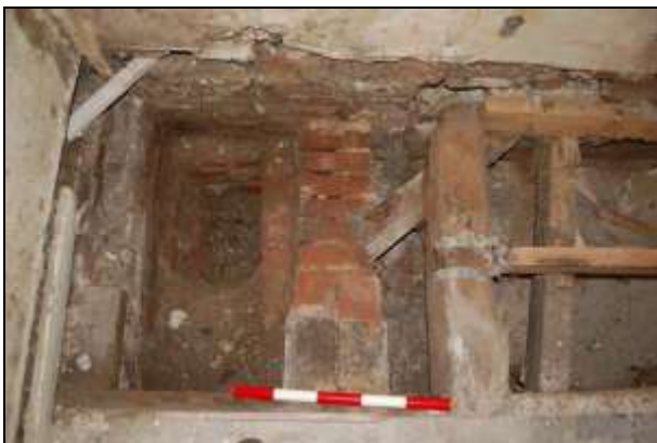
Plate 59: Room G1: exposed southeast corner of the cellar
