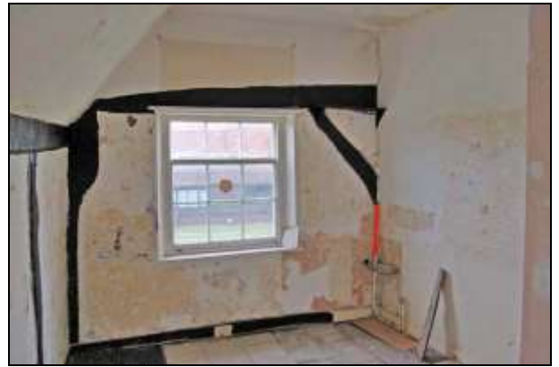
Plate 44: Room F5: north wall
