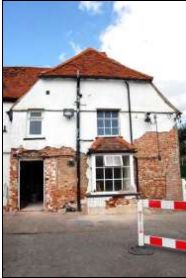
Plate 49: South wall during works
