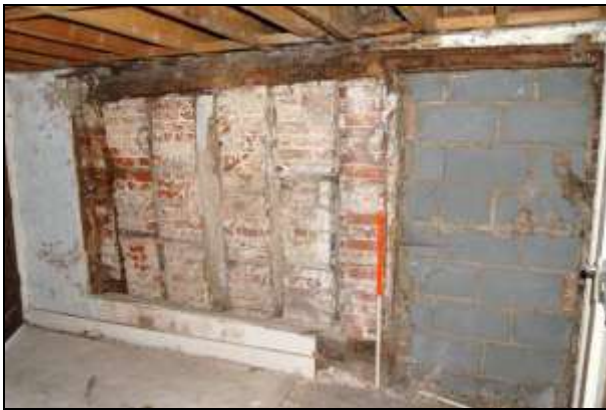
Plate 63: Room G4: exposed west wall
