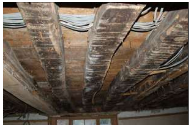
Plate 60: Room G1: ceiling joists
