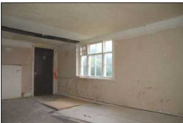
Plate 11: Room G1: northeast corner
