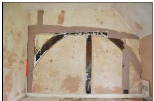
Plate 36: Room F4: north wall
