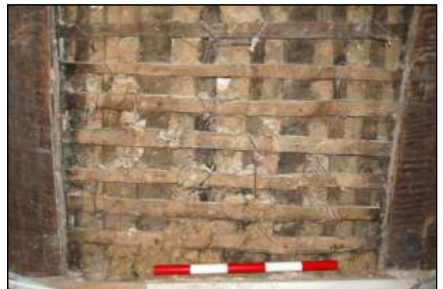
Plate 72: Room F4: north wall detail
