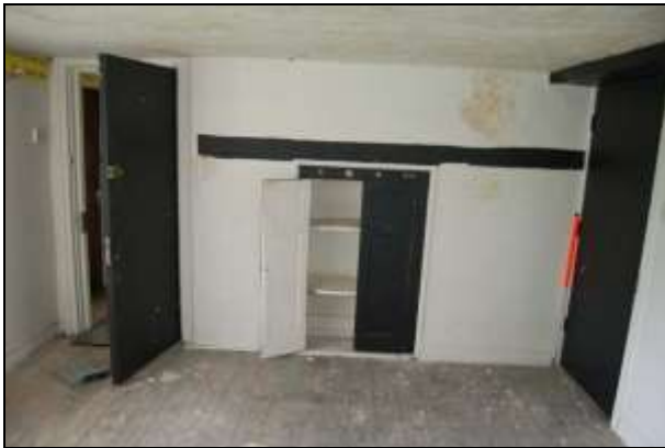
Plate 15: Room G3: south wall
