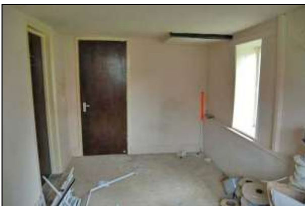
Plate 23: Room G6: south wall
