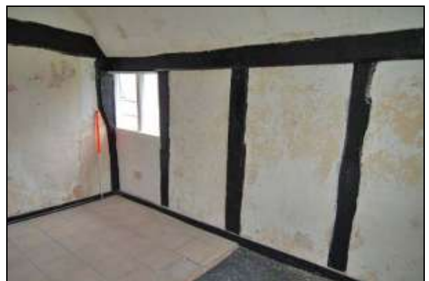
Plate 42: Room F5: southwest corner
