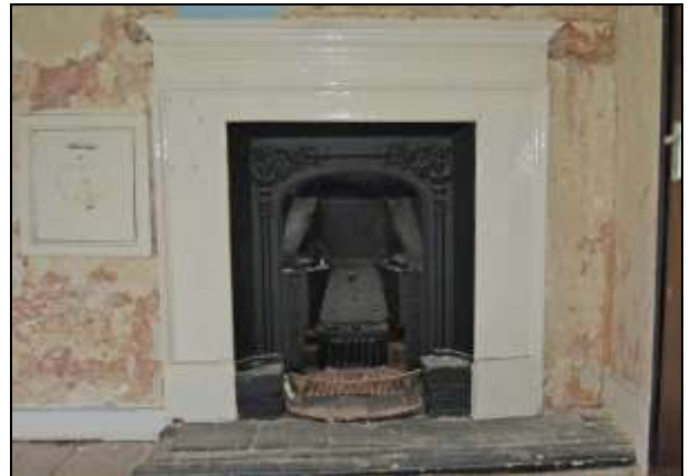
Plate 40: Room F4: fireplace detail
