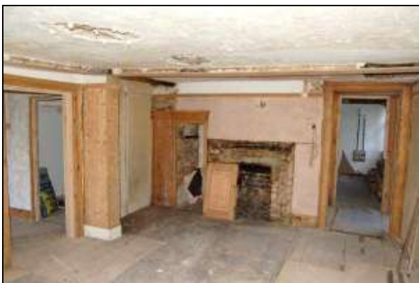
Plate 53: Room G1 looking north
