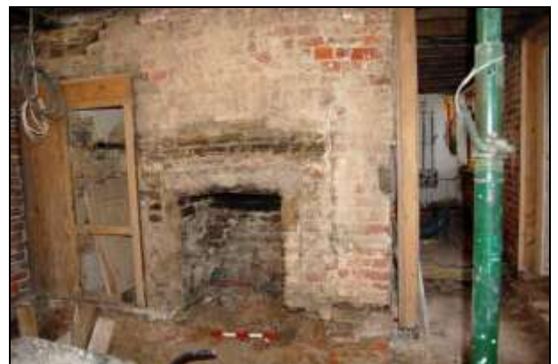
Plate 54: Room G1: fireplace detail
