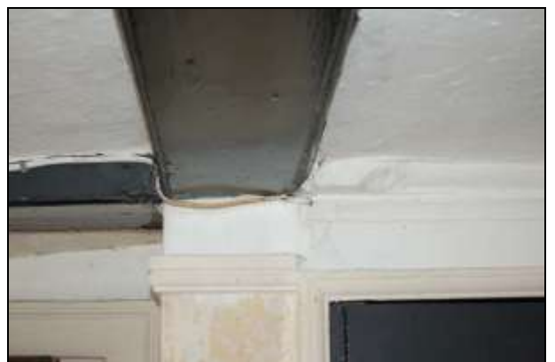
Plate 12: Room G1: beam detail
