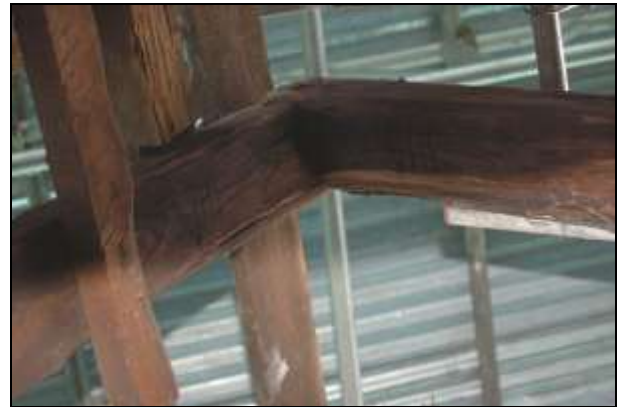
Plate 86: Carpenter's assembly marks
