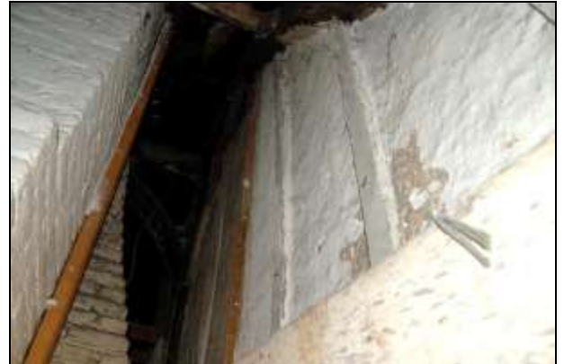
Plate 70: Room F3: studwork in the north wall
