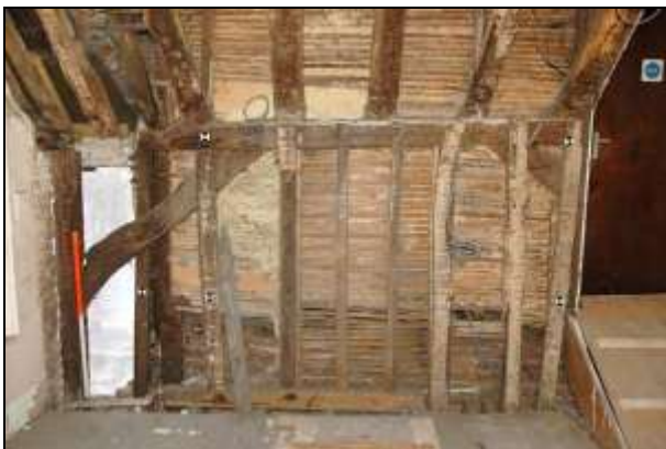
Plate 77: Room F6: west wall
