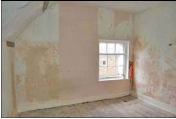
Plate 31: Room F2: south wall
