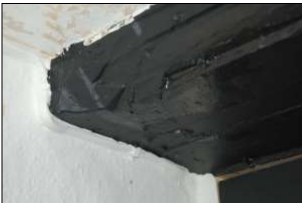
Plate 17: Room G3: chamfer stop detail
