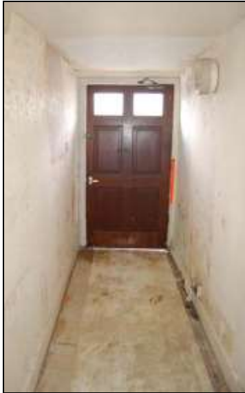
Plate 19: Room G4 looking south
