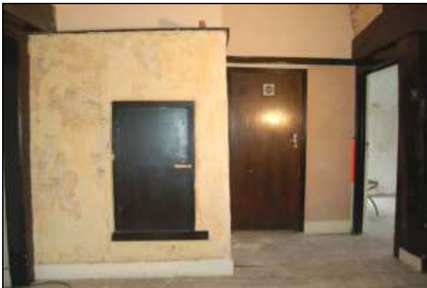
Plate 27: Room F1: east wall
