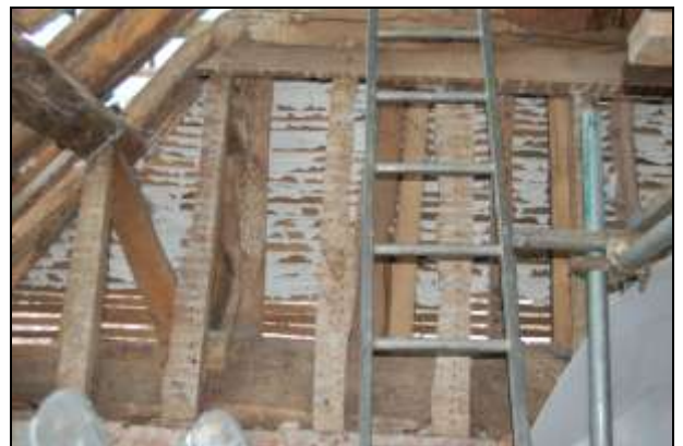
Plate 78: Room F6: double timber frame in the south wall
