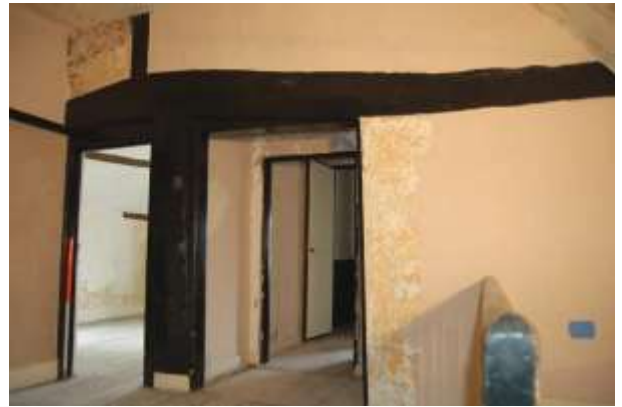
Plate 26: Room F1: south wall
