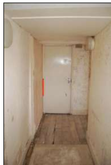
Plate 18: Room G3 looking north
