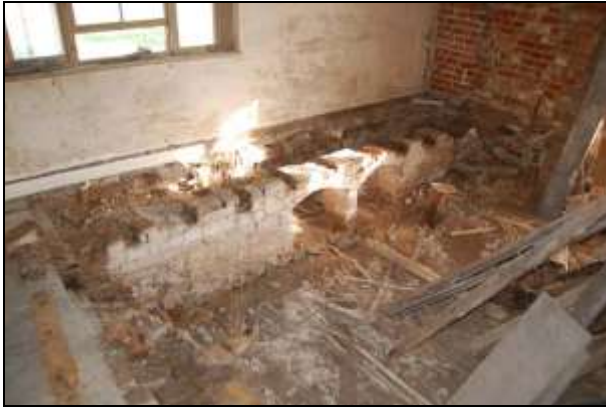
Plate 57: Room G1: exposed western cellar wall
