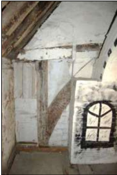
Plate 69: Room F3: south wall
