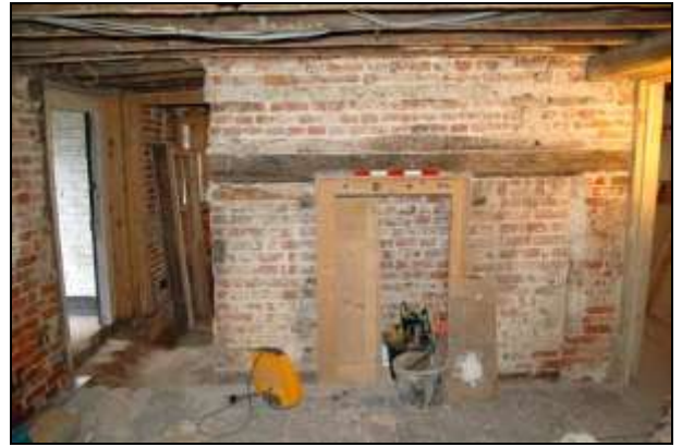
Plate 62: Room G3: exposed south wall
