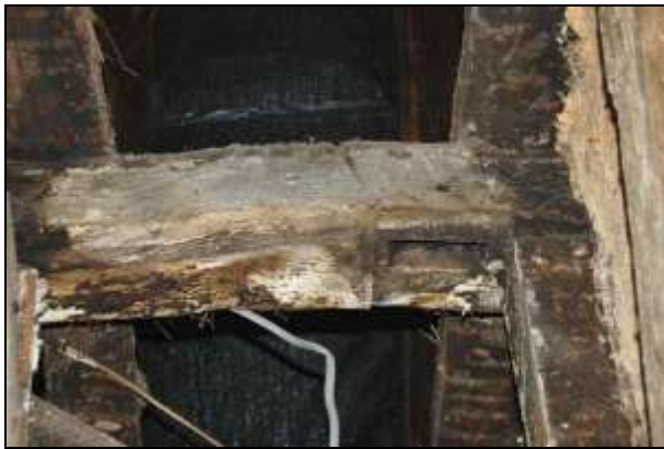
Plate 81: Room F3: scarf joint in the collar purlin
