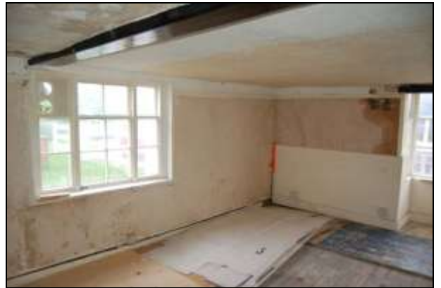
Plate 10: Room G1: southeast corner
