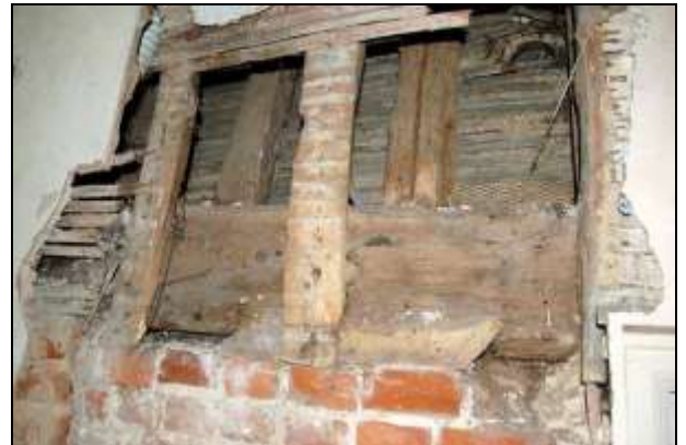
Plate 52: Exposed timberwork in the south wall
