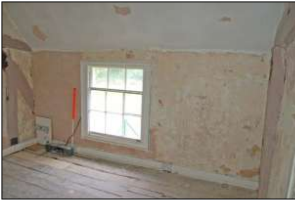
Plate 37: Room F4: east wall
