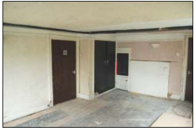
Plate 8: Room G1: northwest corner
