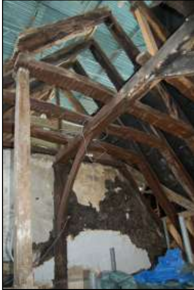
Plate 79: Room F3: crown post & collar purlin
