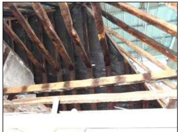
Plate 84: Room F4: collar purlin
