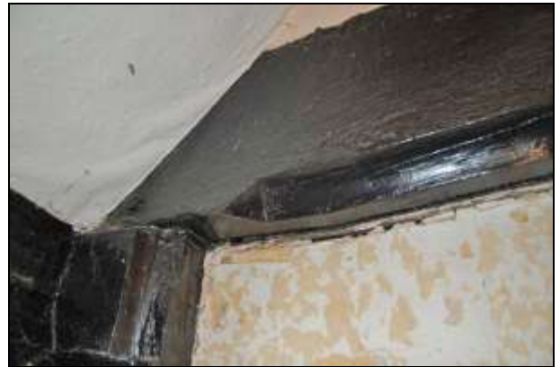
Plate 28: Room F1: chamfer stop detail
