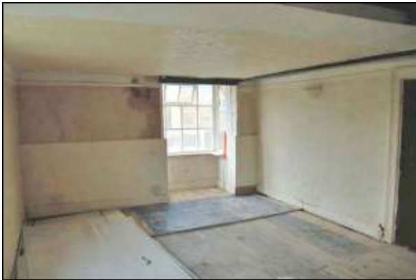
Plate 9: Room G1: southwest corner
