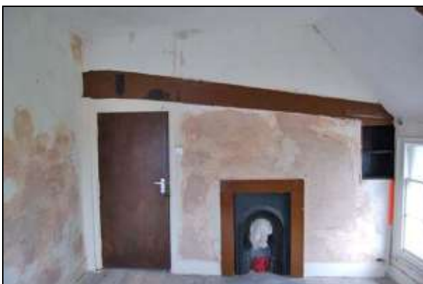
Plate 29: Room F2: north wall
