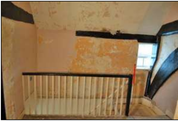
Plate 25: Room F1: west wall
