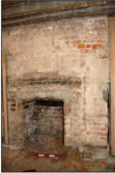
Plate 55: Room G1: fireplace detail
