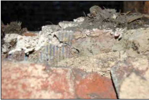
Plate 73: Room F4: wallpaper remains in east wall
