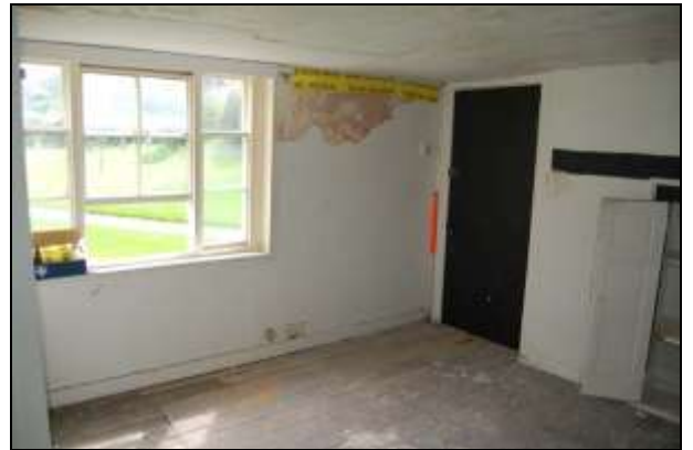
Plate 16: Room G3: southeast corner
