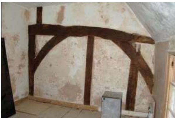
Plate 71: Room F4: north wall
