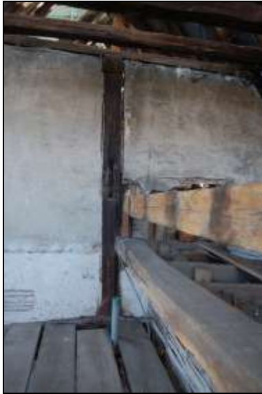
Plate 85: Room F4: crown post & collar purlin
