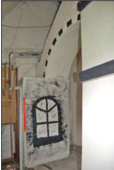
Plate 33: Room F3 looking southwest
