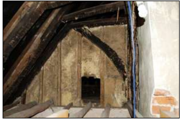
Plate 80: Room F1: studwork in the north wall
