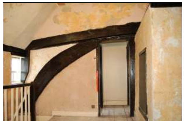
Plate 24: Room F1: north wall
