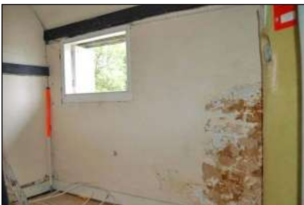
Plate 35: Room F3: east wall
