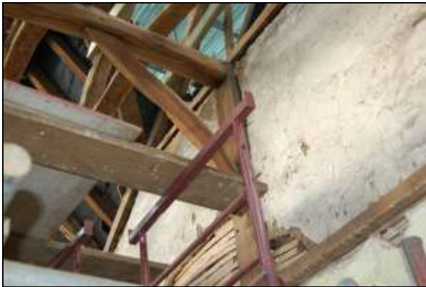
Plate 87: Room F2: crown post & collar purlin
