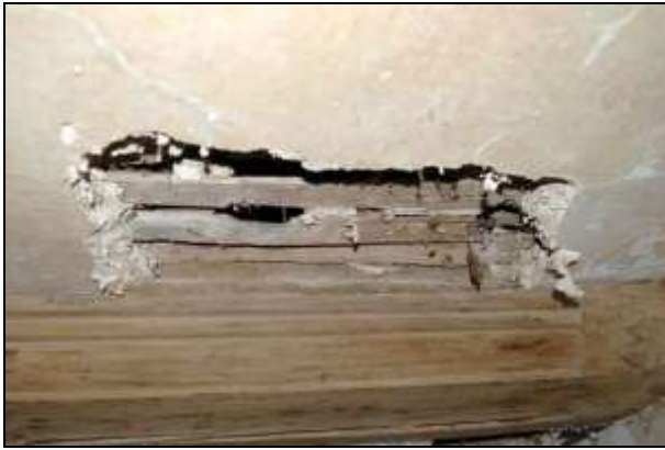
Plate 61: Room G3: spinal beam, chamfer stop and lath and plaster
