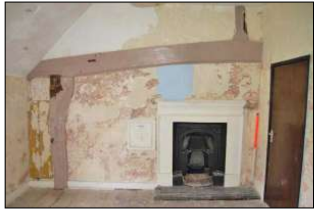
Plate 38: Room F4: south wall
