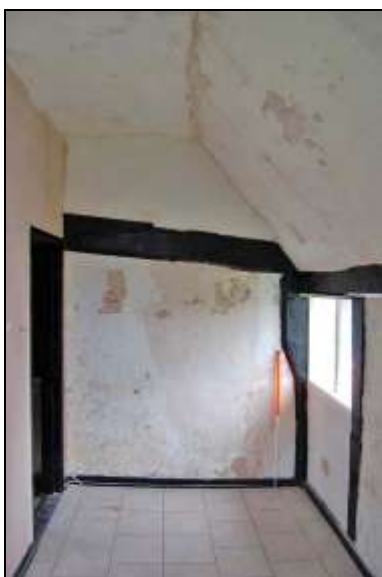
Plate 41: Room F5: south wall
