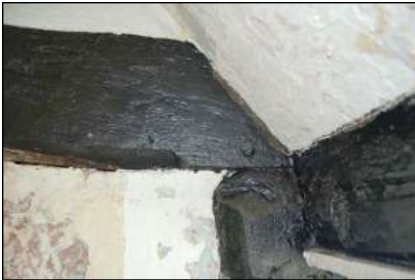
Plate 45: Room F5: tiebeam chamfer detail
