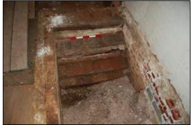
Plate 58: Room G5: exposed cellar stairs
