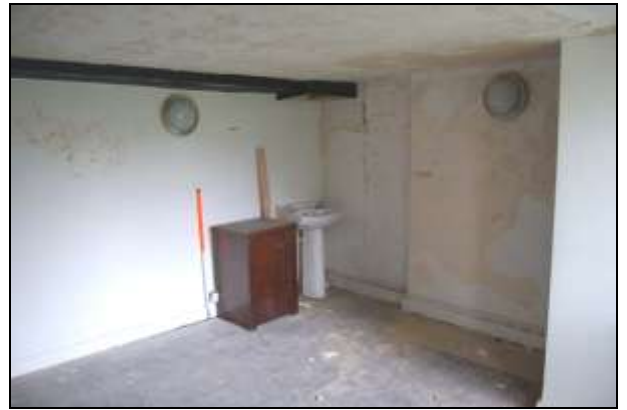
Plate 14: Room G3: northwest corner
