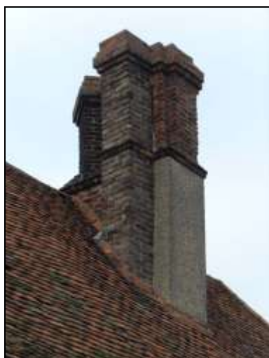
Plate 47: Central chimney stack
