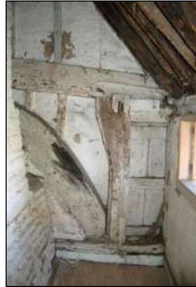
Plate 68: Room F3: north wall
