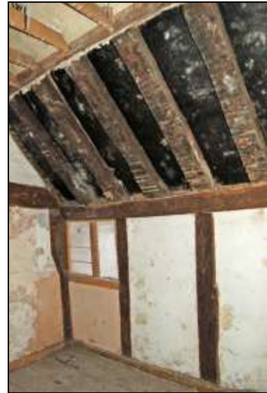
Plate 76: Room F5: exposed rafters
