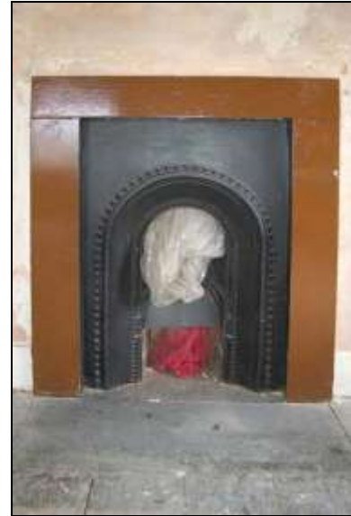
Plate 32: Room F2: fireplace detail
