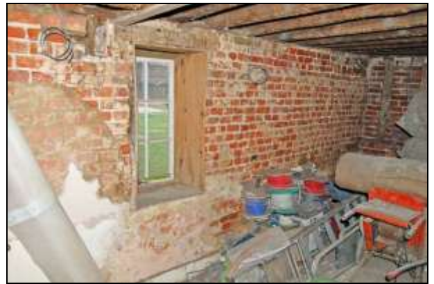
Plate 64: Room G6: exposed west wall
