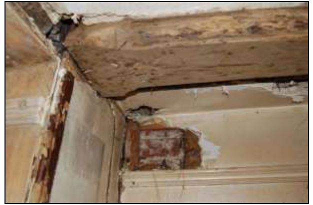
Plate 56: Room G1: chamfer stop in binding beam
