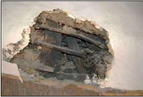
Plate 67: Room F1: blackened wattle & daub in south wall
