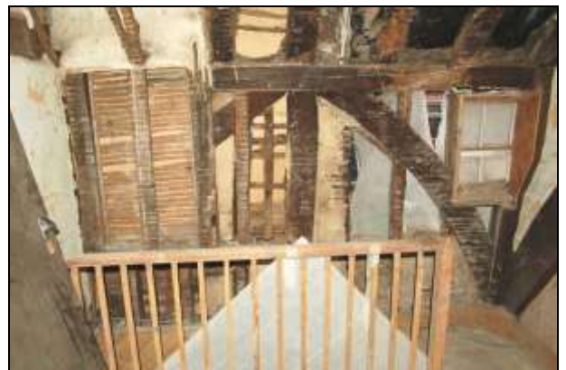
Plate 66: Room F1: west wall
