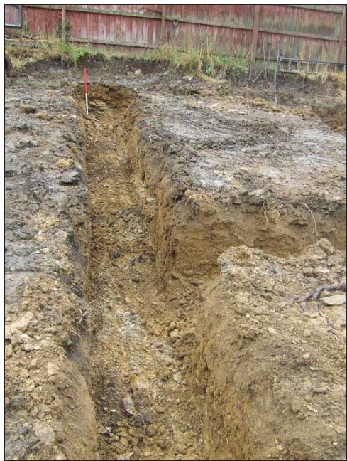
Plate 5: Footing trench towards middle of site, looking east, 1m scale
