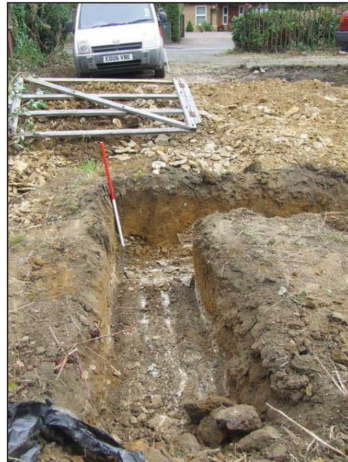
Plate 2: Footing trench in south eastern corner, looking south, 1m scale
