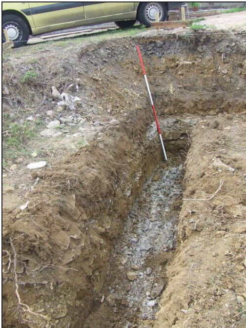
Plate 1: Footing trench in reduced area, looking south west, 2m scale
