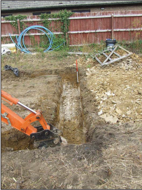
Plate 3: Southernmost footing trench, looking east, 1m scale
