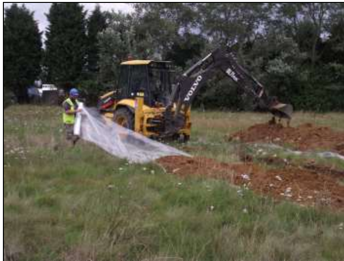
Plate 2: Laying of protective polythene sheeting in the MG5 grass area.
