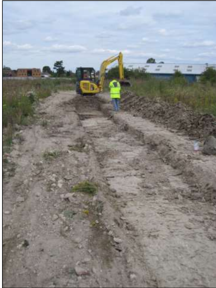
Plate 1: General view, excavating Trench 3
