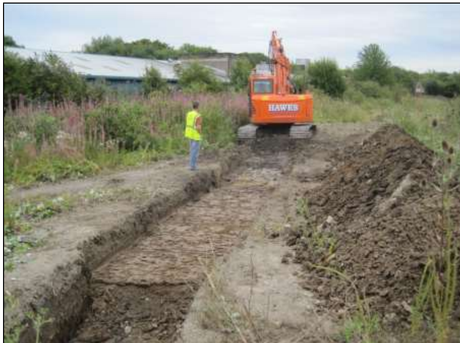
Plate 2: General view, excavating Trench 4
