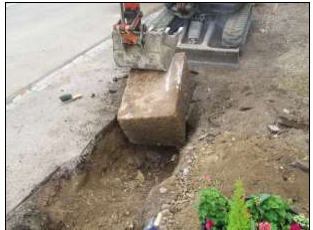
Plate 2: Removing the stones
