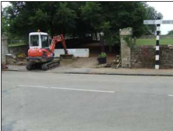
Plate 1: Entrance prior to removal of foundations
