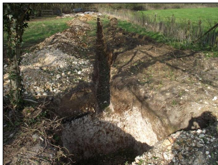
Plate 3: Soakaway and service trench, looking NW
