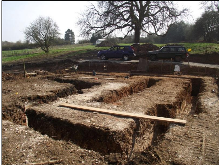
Plate 1: Footing trenches, looking SE
