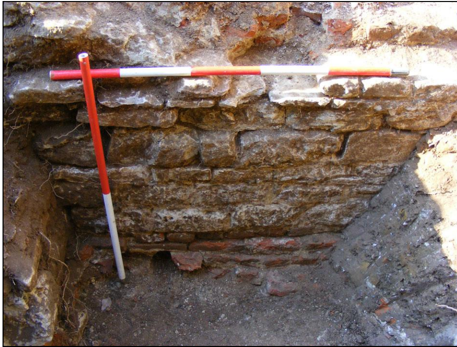
Plate 17: Detail of external clunch facing (007) on east elevation, structure 006, facing west
