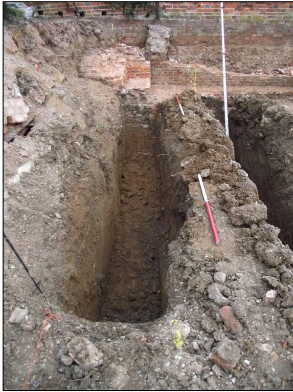
Plate 3: Footing B 'cartshed' area, facing north
