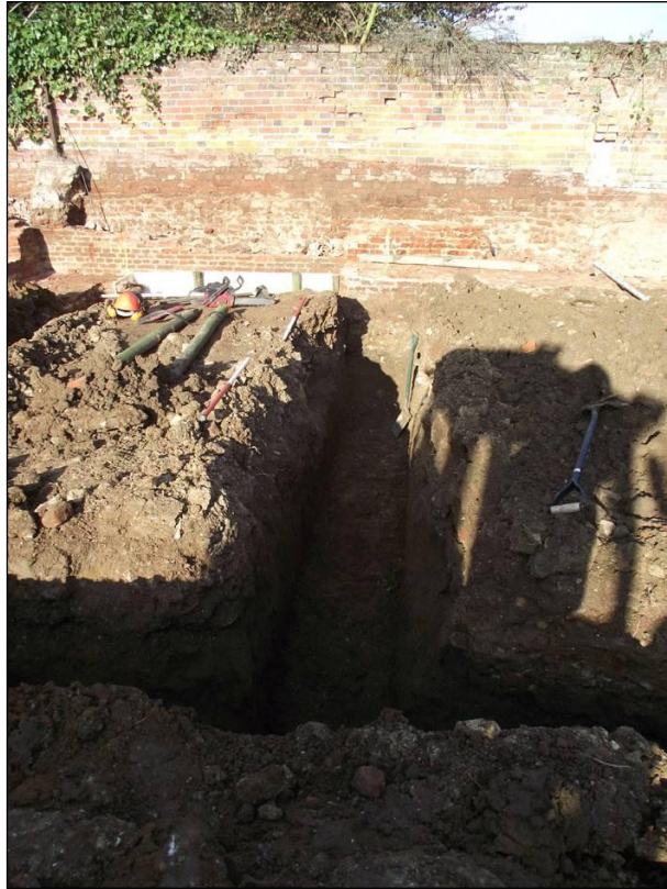
Plate 7: Footing D, facing west
