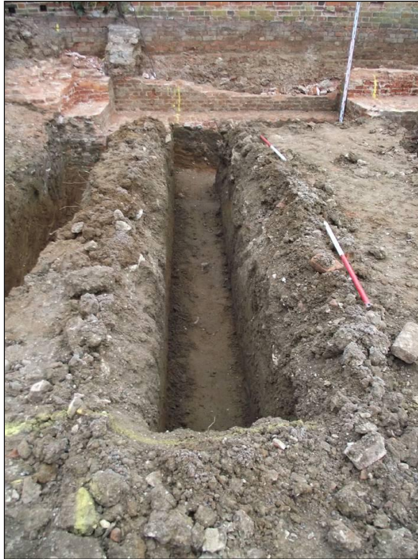
Plate 5: Footing C, facing north
