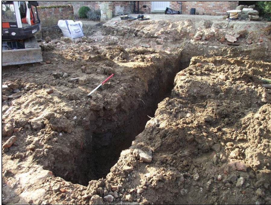
Plate 9: Footing F, facing south-west
