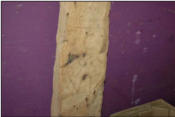
Plate 15: Detail of graffiti on south post of Truss 1
