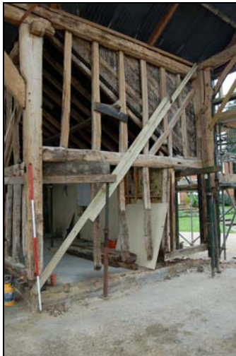
Plate 27: North midstrey, looking north west, 2m scale
