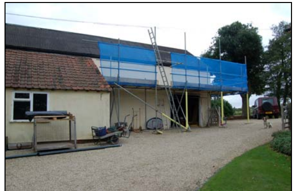
Plate 6: Exterior of barn, looking south east, 2m scale
