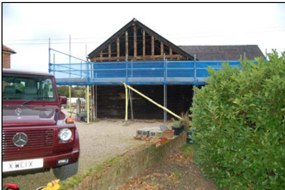
Plate 5: Exterior of barn, looking east, 2m scale
