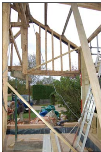
Plate 35: Aisle, looking east, 2m scale
