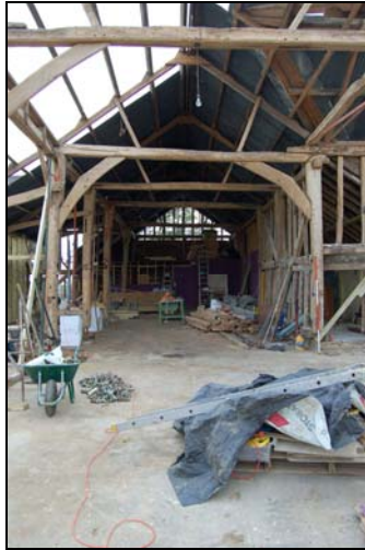
Plate 25: Truss 4, looking west, 2m scale
