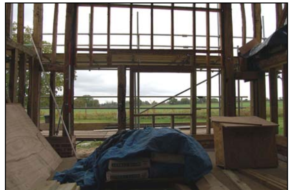
Plate 18: South midstrey/Bay 2, looking south, 2m scale
