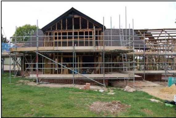
Plate 3: Exterior of barn, looking north, 2m scale
