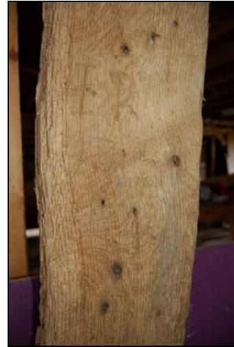
Plate 14: Detail of graffiti on south post of Truss 1
