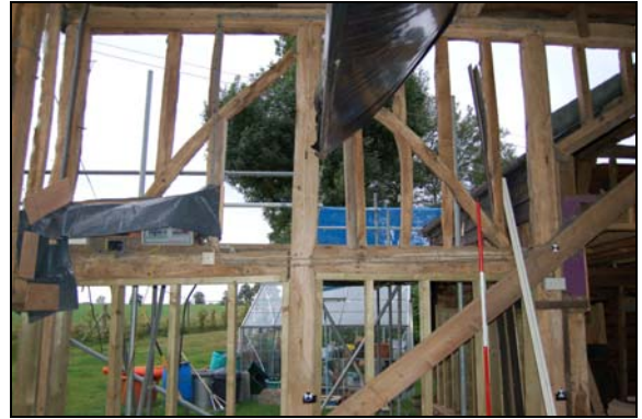
Plate 20: South midstre, looking west, 2m scale
