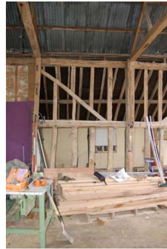
Plate 22: Bay 3, looking north, 2m scale
