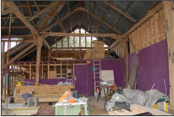
Plate 13: Truss 1, looking west, 2m scale
