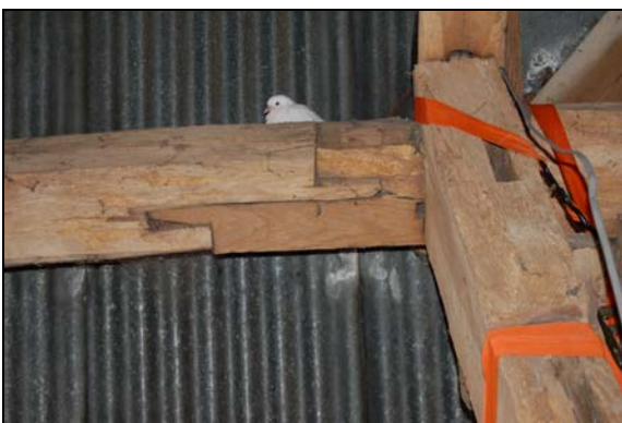
Plate 23: Counter bladed scarf joint on southern side of Bay 2
