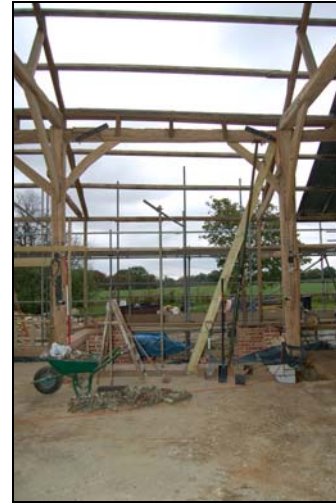
Plate 8: Bay 5, looking south, 2m scale
