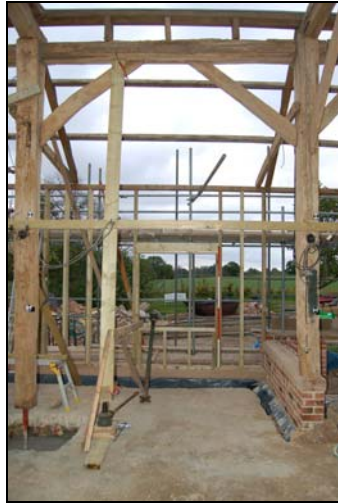
Plate 7: Bay 6, looking south, 2m scale
