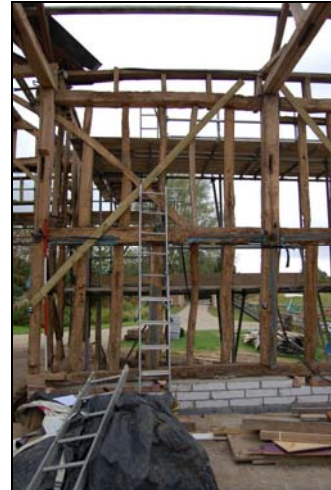
Plate 32: Bay 6, looking north, 2m scale
