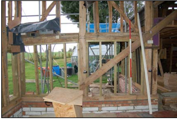
Plate 19: South midstre, looking west, 2m scale
