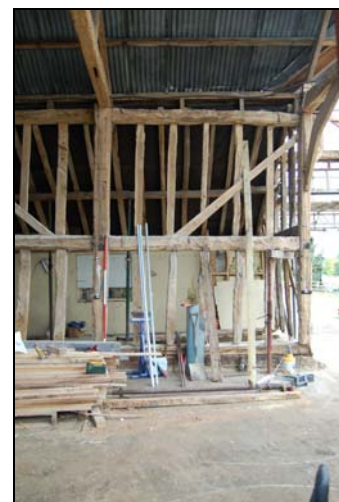
Plate 24: Bay 4, looking north, 2m scale
