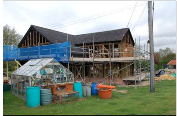
Plate 4: Exterior of barn, looking north east, 2m scale
