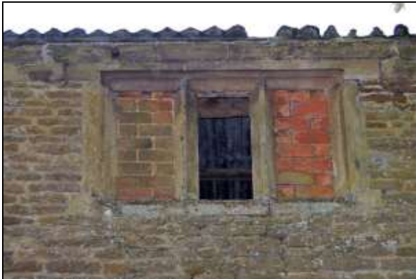
Plate 9: Window 2, upper floor
