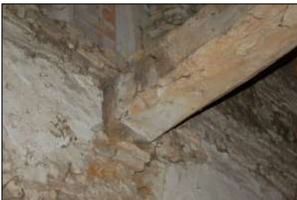
Plate 29: Lambs tongue chamfer stop
