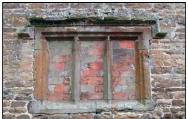
Plate 12: Window 5, ground floor
