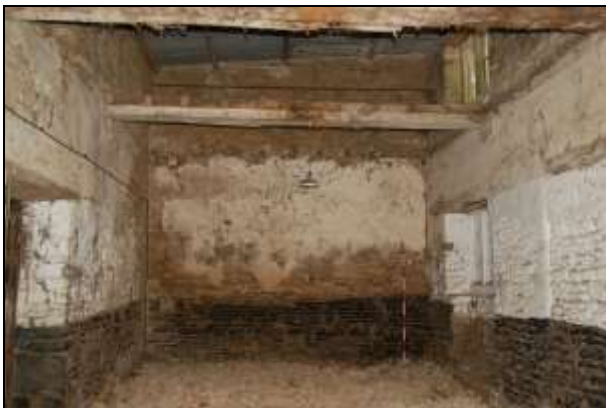
Plate 15: Interior looking north
