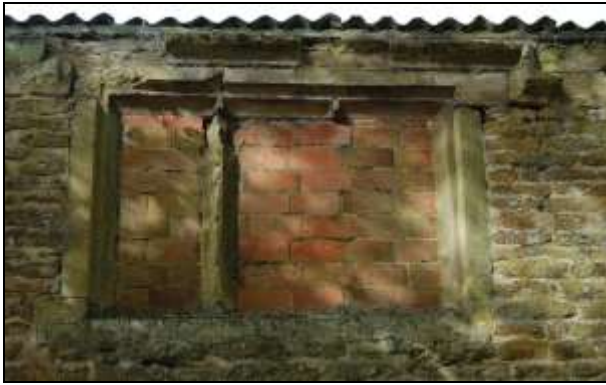
Plate 7: Window 1, upper floor
