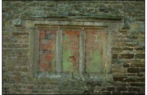
Plate 8: Window 2, ground floor
