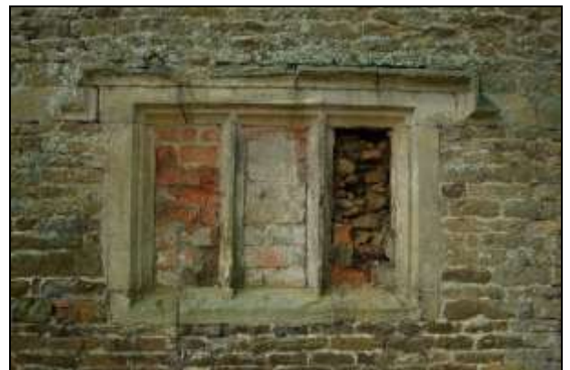
Plate 6: Window 1, ground floor
