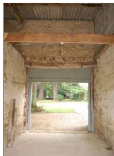
Plate 30: Carriageway looking east
