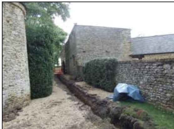
Plate 33: Drainage trench alongside outbuilding, looking south southwest
