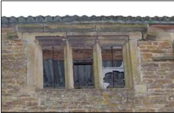
Plate 13: Window 5, upper floor
