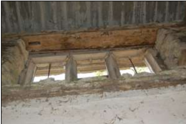
Plate 27: Lintels over Window 5, upper level
