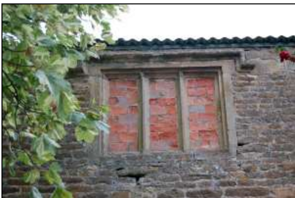
Plate 11: Window 4, upper floor
