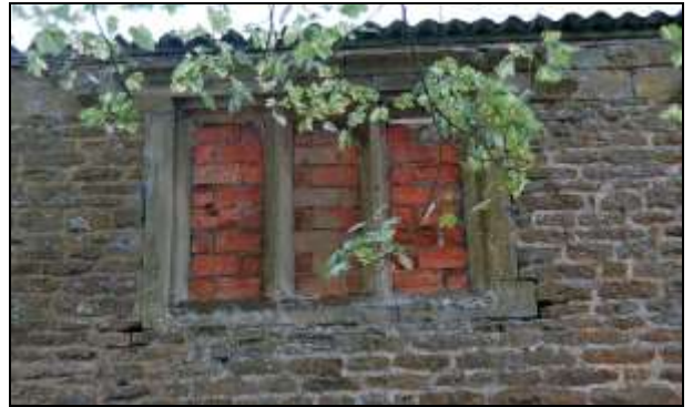
Plate 10: Window 3, upper floor
