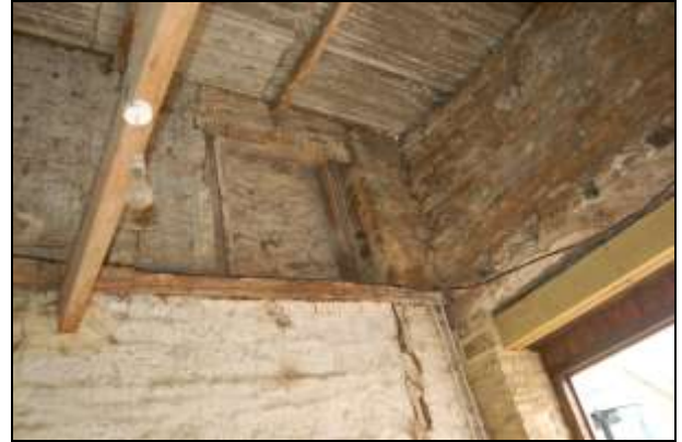
Plate 32: Blocked opening in south wall of carriageway
