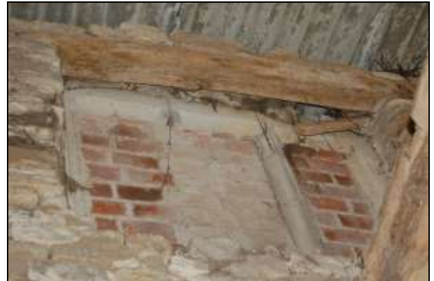
Plate 28: Lintel over Window 1, upper level
