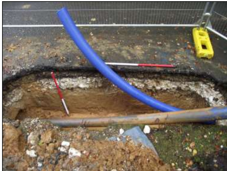
Plate 6: Main 3 – example of stratigraphy (Tr 53), looking N (scale 2×1m)
