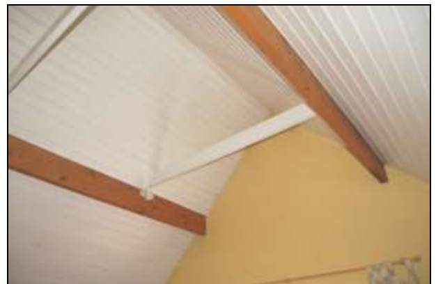
Plate 48: Room F0 ceiling, looking west.
