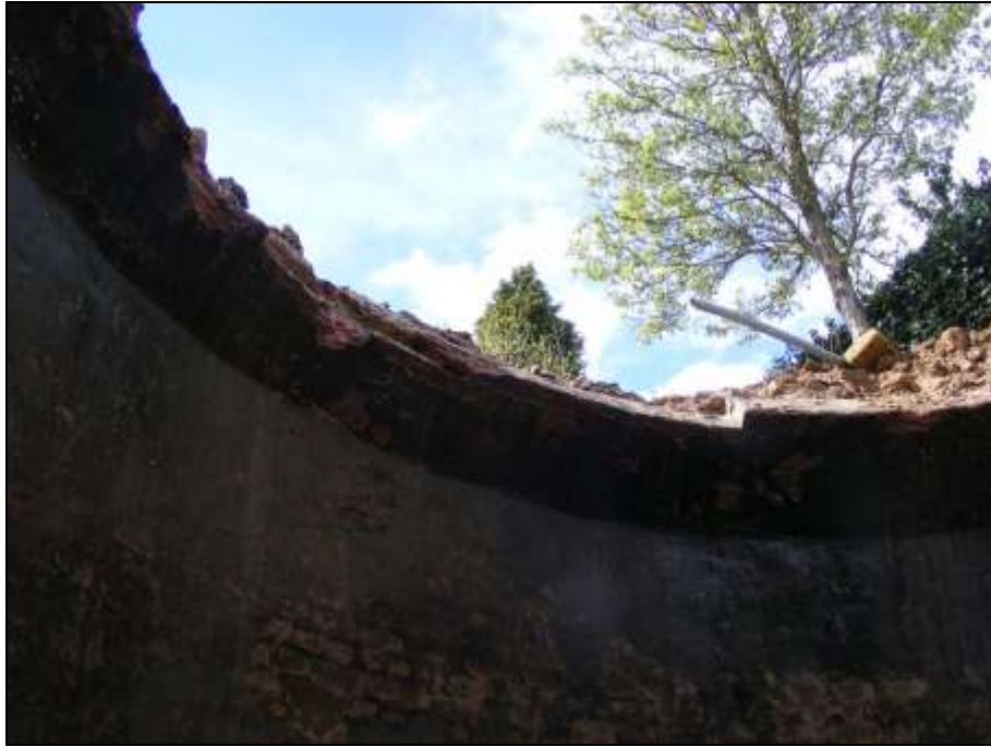
Plate 56: View from the bottom of the cistern
