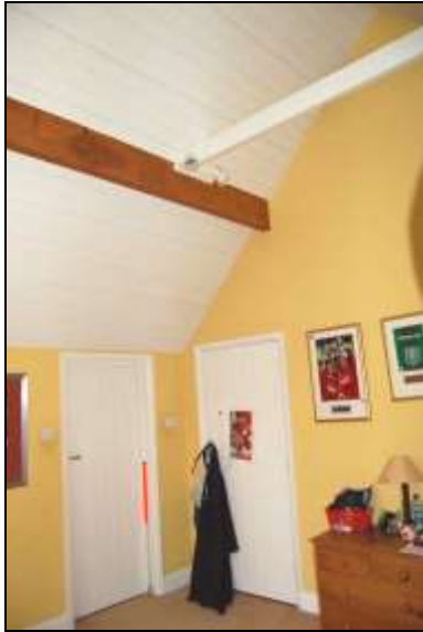
Plate 49: Room F9: southeast corner.
