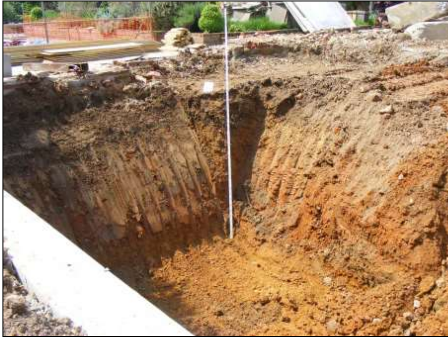
Plate 54: Ground reduction for the cellar
