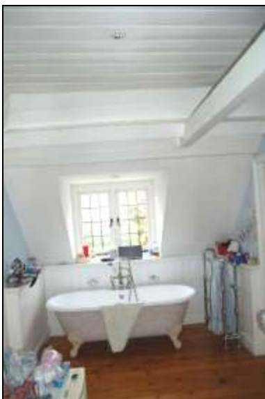
Plate 41: Room F5, west wall.
