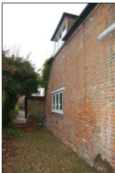
Plate 5: East elevation, looking southwest.
