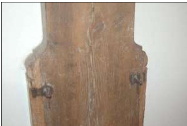
Plate 17: Room G2: detail of moulding and metal stops.
