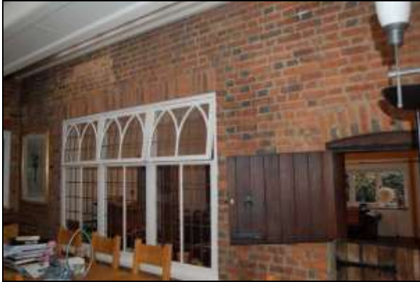
Plate 31: Room G10, looking northeast.
