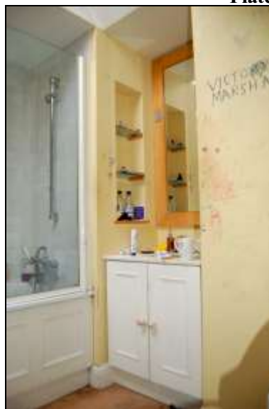
Plate 53: Bathroom 2 (F12), looking northeast.
