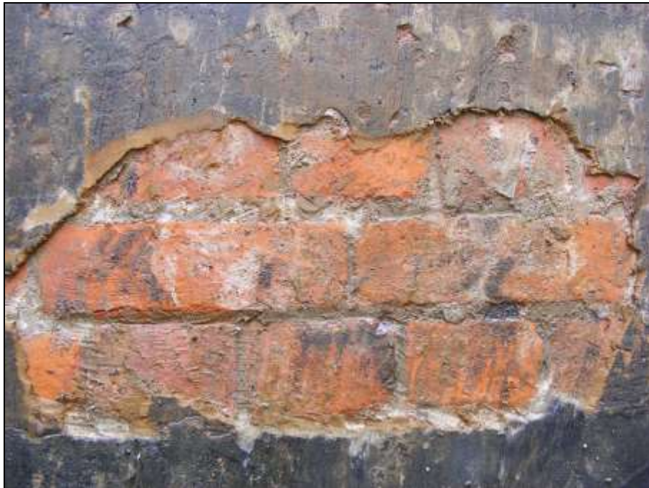
Plate 57: Detail of the cistern walls
