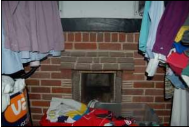
Plate 25: Laundry room (G5), detail in south wall.
