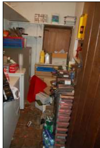
Plate 24: Room G4 looking south.
