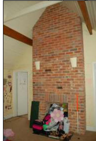
Plate 52: Room F11: north wall.
