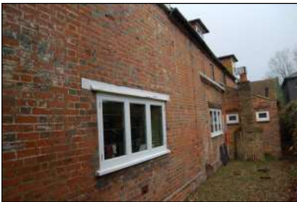
Plate 3: East elevation, looking north-northwest.
