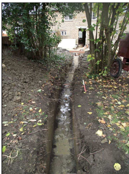
Plate 3: Drainage trench, looking SW (scale 1m)
