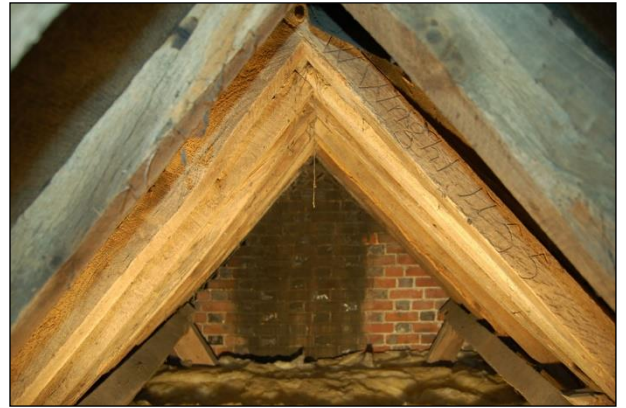
Plate 50: Roof over F3 looking south
