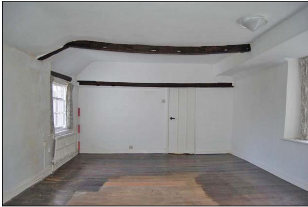
Plate 37: Room F3: south wall
