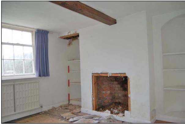
Plate 13: Room G2: southeast corner
