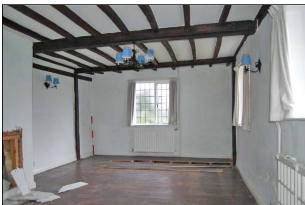
Plate 23: Room G5: east wall
