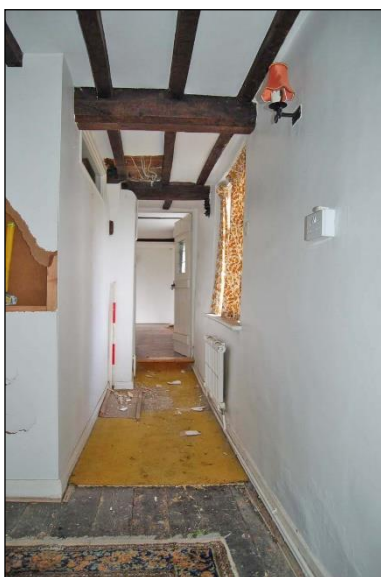
Plate 11: Room G1: passage to Room G4
