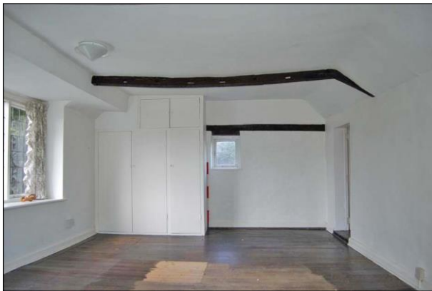
Plate 39: Room F3: north wall
