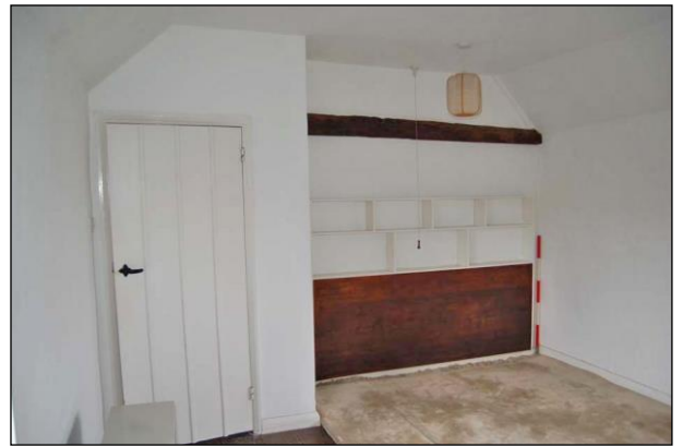
Plate 44: Room F6: north wall
