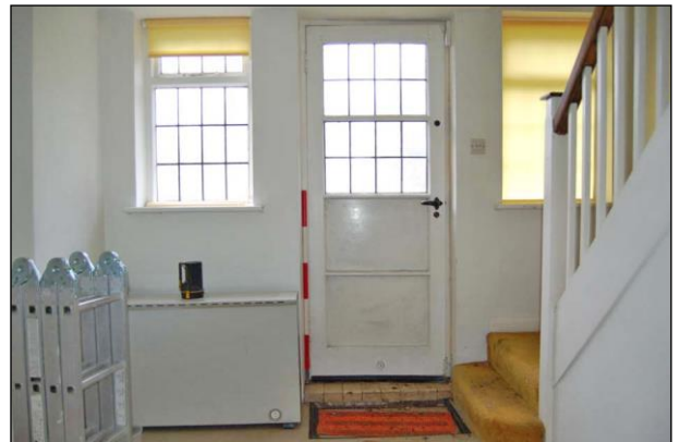
Plate 28: Room G7: west wall
