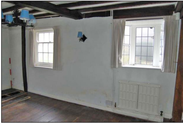
Plate 25: Room G5: south wall
