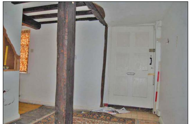
Plate 10: Room G1: southeast corner
