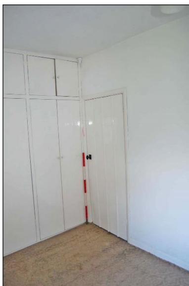
Plate 41: Room F4: southwest corner
