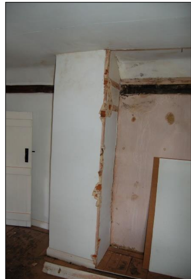
Plate 58: Room F2 north wall
