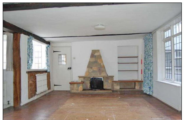
Plate 18: Room G4: south wall
