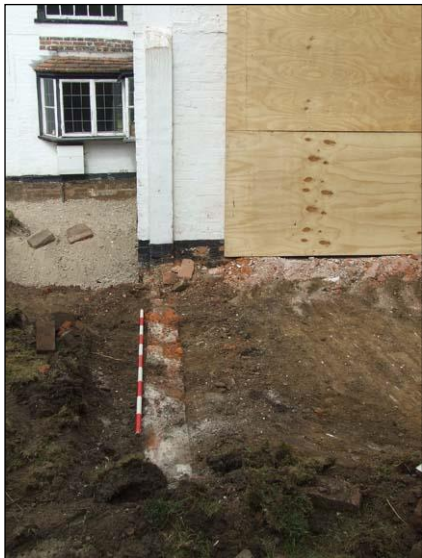
Plate 65: South wall of crosswing
