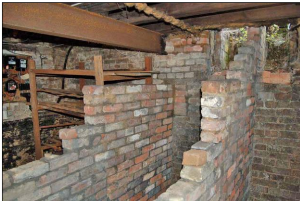
Plate 9: Cellar: looking northeast
