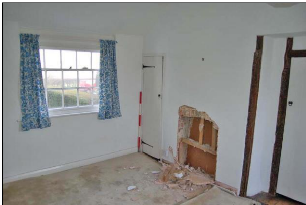
Plate 45: Room F6: southeast corner
