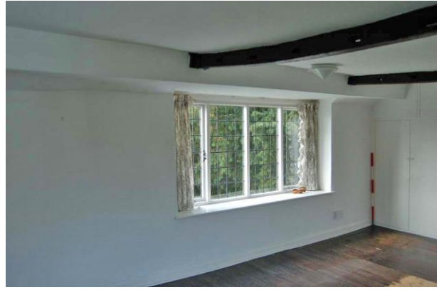
Plate 40: Room F3: northwest corner
