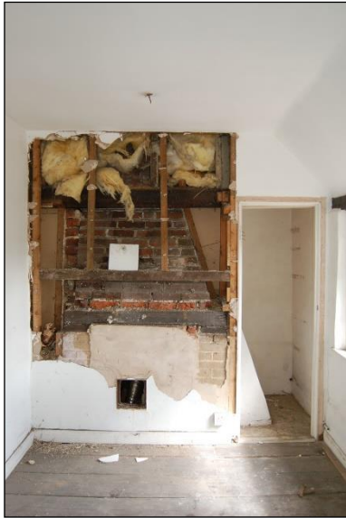
Plate 61: Room F4: chimney breast
