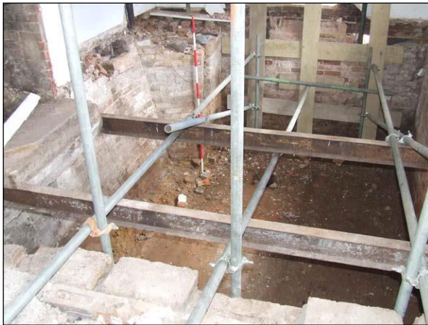
Plate 57: Room G5: cellar below the floor
