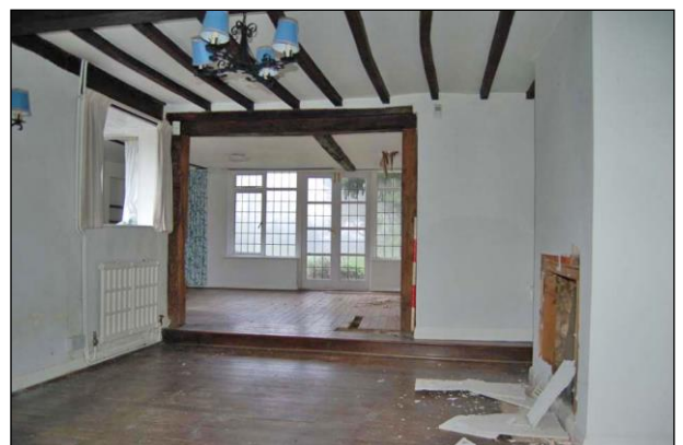
Plate 24: Room G5: west wall
