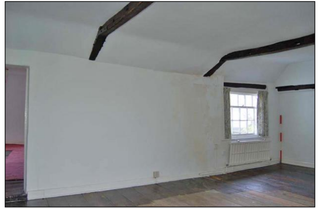
Plate 38: Room F3: east wall
