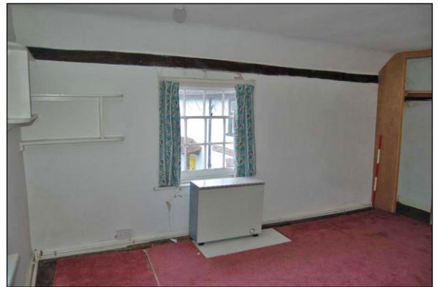
Plate 34: Room F2: south wall
