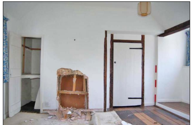
Plate 46: Room F6: south wall
