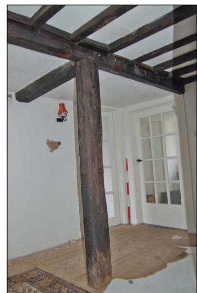
Plate 12: Room G1: southwest corner
