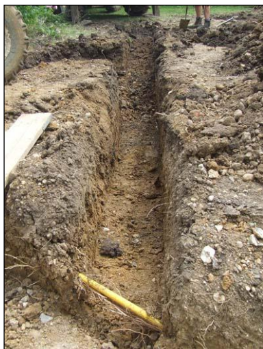
Plate 67: Service trench east of the house
