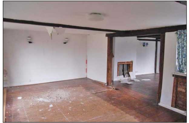
Plate 20: Room G4: looking northeast
