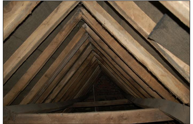
Plate 52: Roof over crosswing looking east
