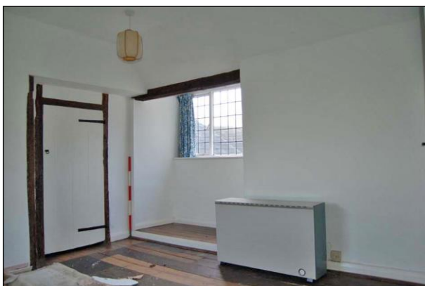
Plate 47: Room F6: southwest corner
