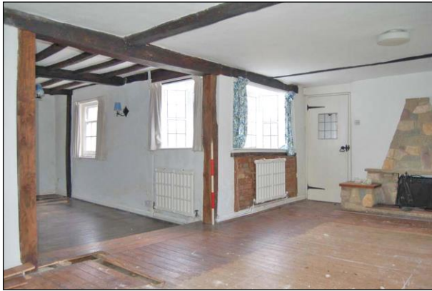
Plate 19: Room G4: looking southeast
