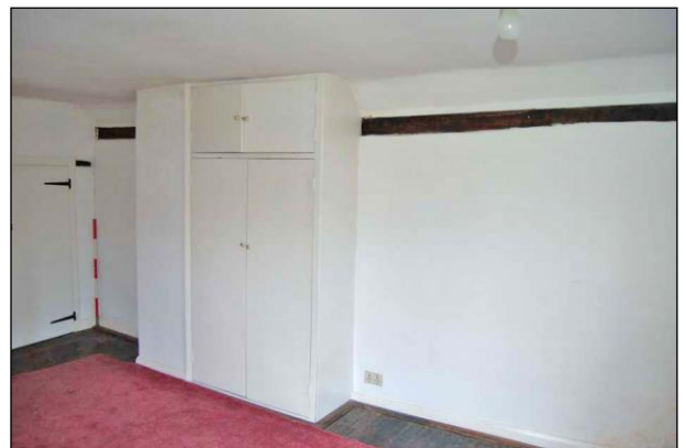
Plate 36: Room F2: north wall
