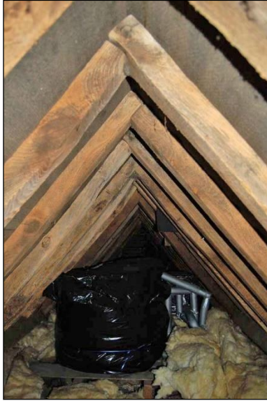
Plate 49: Roof over main range looking south
