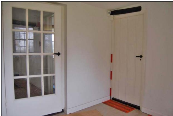
Plate 27: Room G7: southeast corner
