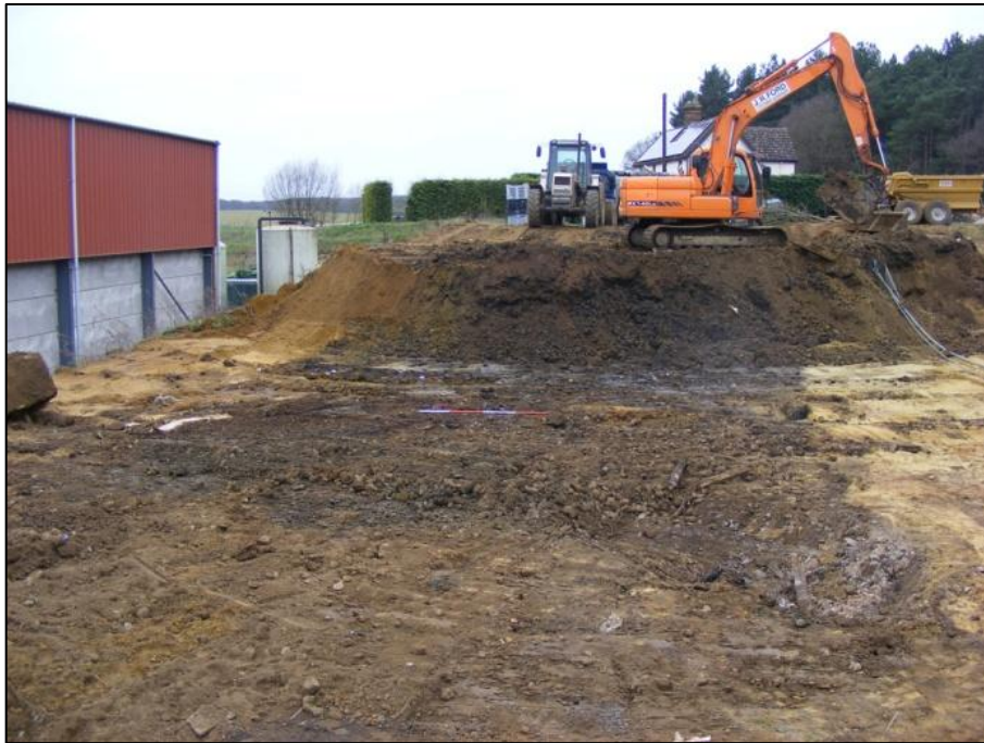
Plate 3: Large modern pit at south edge of development area, facing west
