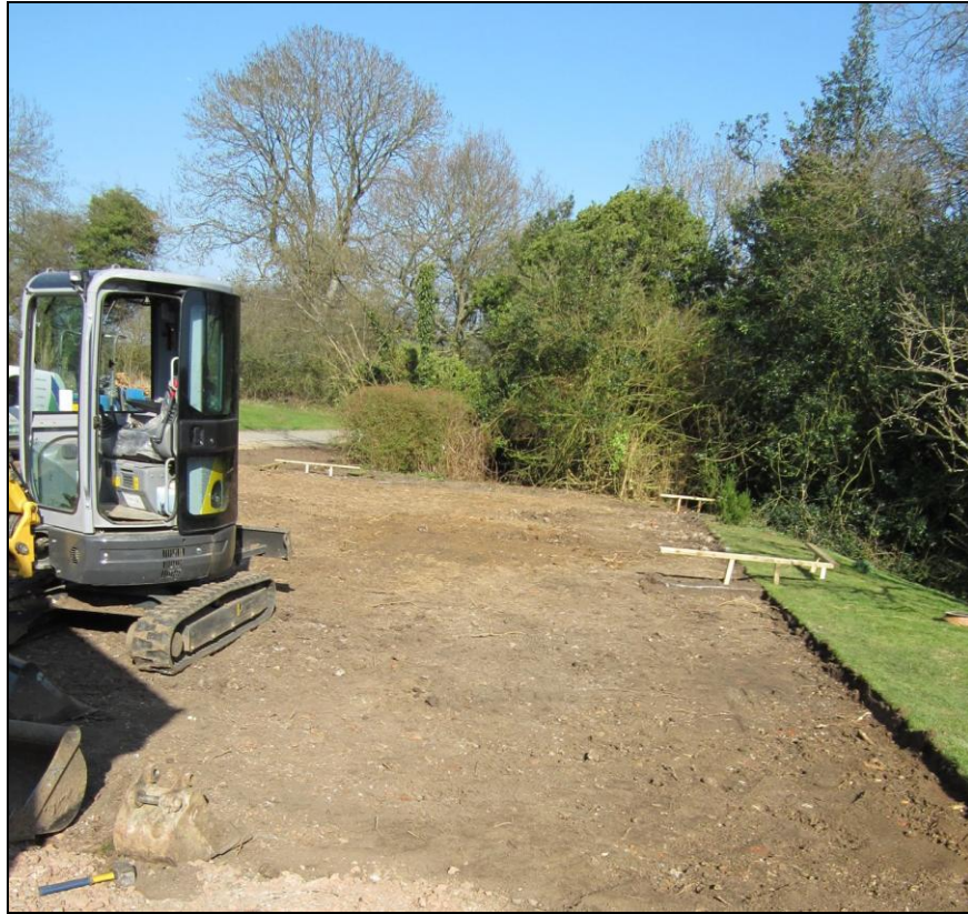
Plate 1: South side of site after stripping
