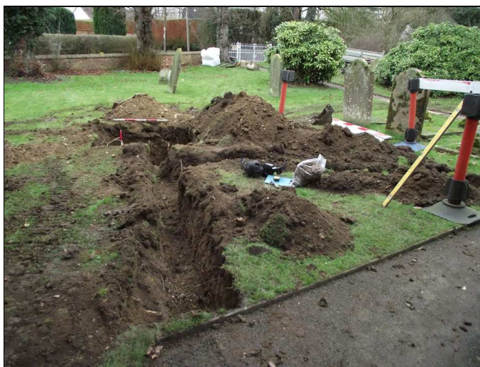
Plate 6: Soakaway 3 and associated drainage gullies, looking north-west ( scale 1m )
