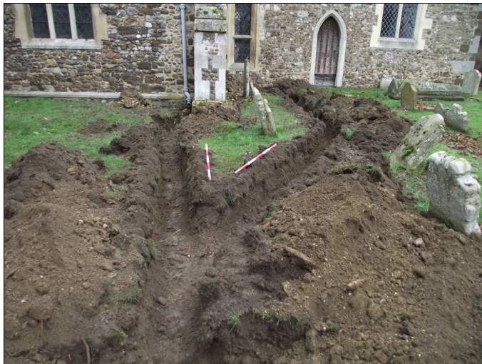
Plate 2: Drainage gullies associated with Soakaway 1, looking N ( scale 2×1m )
