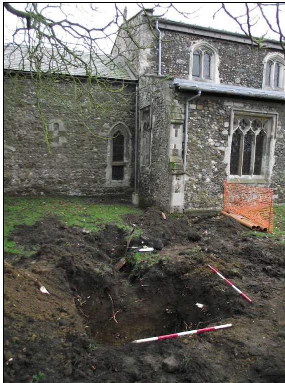
Plate 8: Soakaway 4, looking south ( scale 2×1m )
