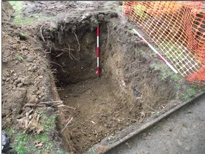
Plate 4: Soakaway 2, looking NW ( scale 2×1m )
