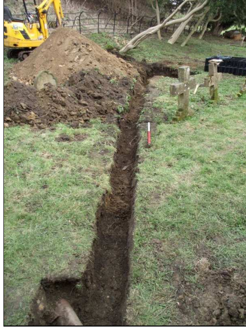
Plate 5: Drainage gully associated with Soakaway 2, looking SE ( scale 1m )
