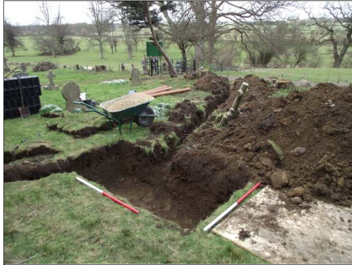
Plate 7: Soakaway 3 and associated drainage gullies, looking NW ( scale 2×1m )
