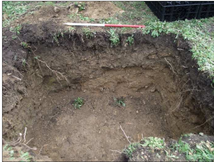
Plate 6: Soakaway 2, looking SE ( scale 1m )
