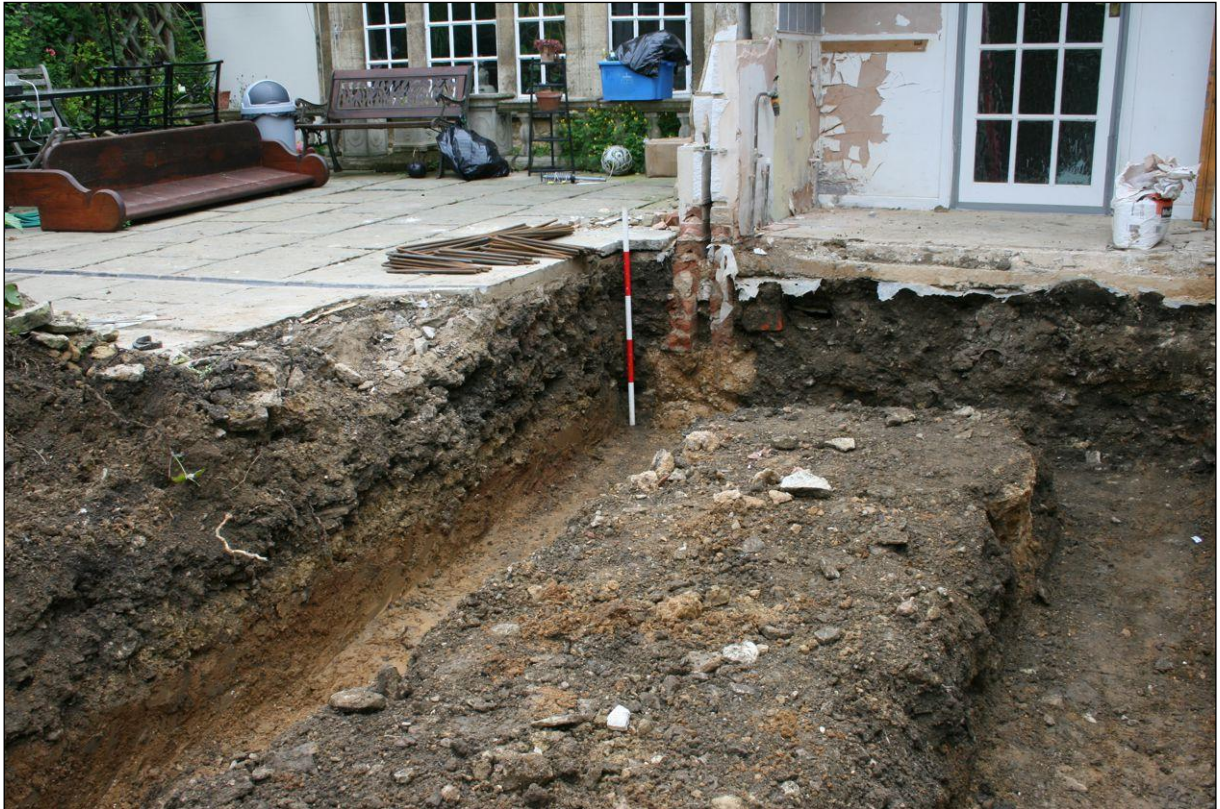
Plate 1: Extension footings, looking north-east
