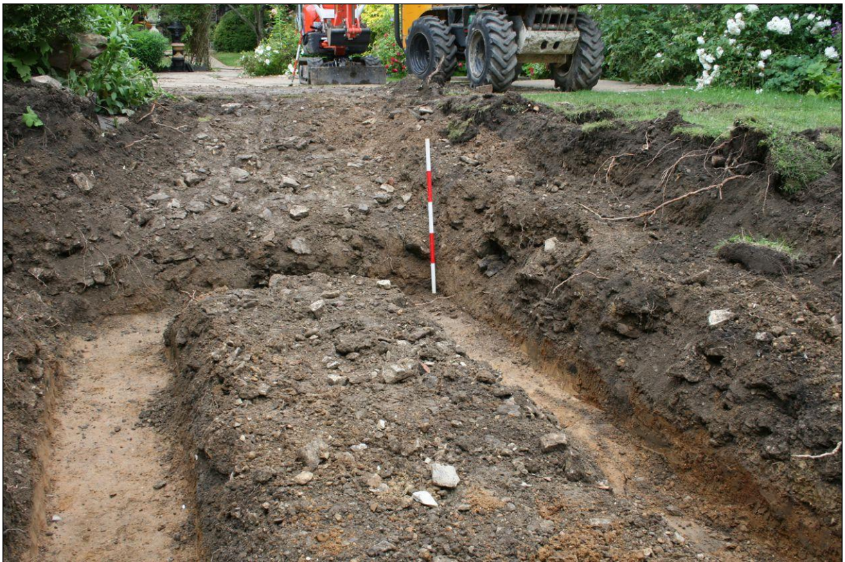
Plate 2: Extension footings, looking north-west
