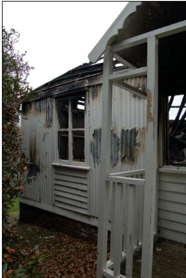
Plate 3: Building 1; west end of south elevation
