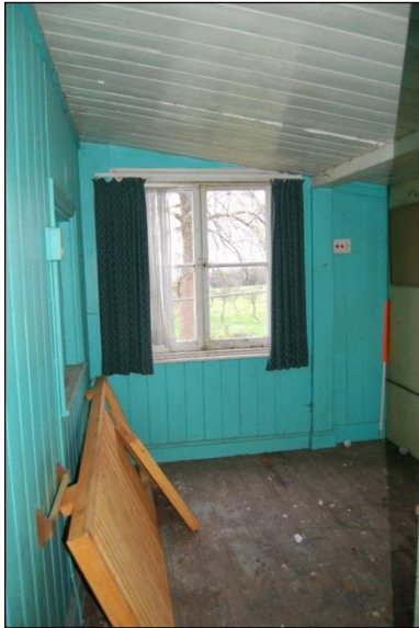
Plate 19: Room G3; north wall
