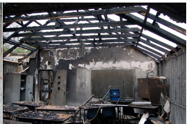
Plate 30: Room G9; west wall
