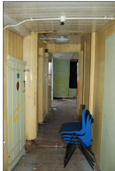
Plate 16: Room G2; looking west
