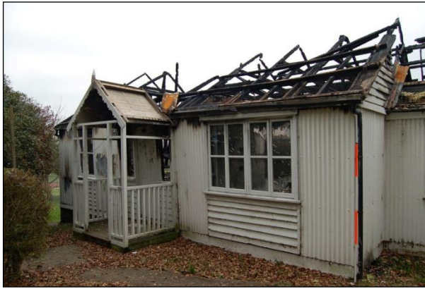
Plate 1: Building 1; south elevation
