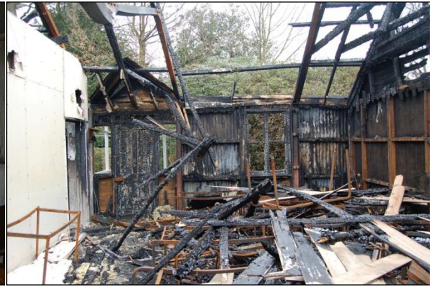
Plate 26: Room G8 looking south
