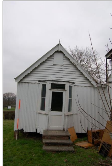
Plate 4: Building 2; south elevation
