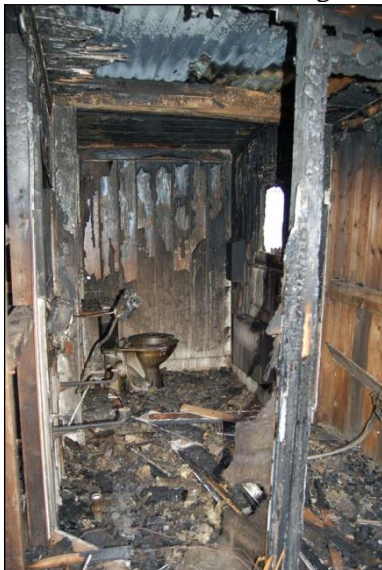
Plate 23: Room G6 looking north
