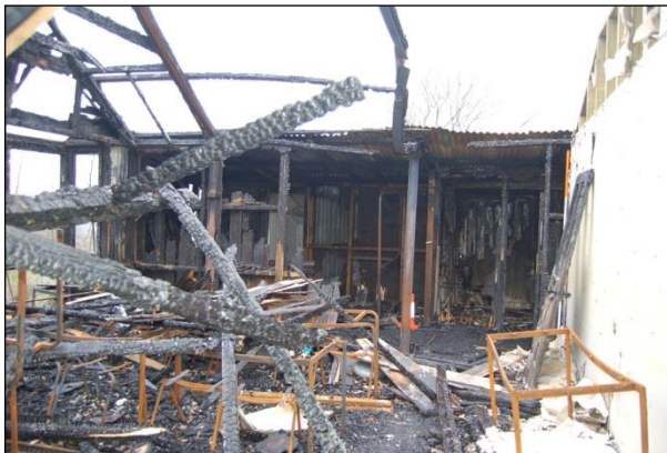
Plate 27: Room G8 looking north
