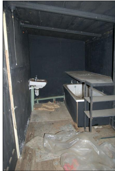
Plate 20: Room G4; north wall
