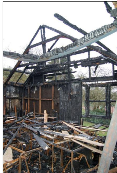
Plate 28: Room G8 looking southwest
