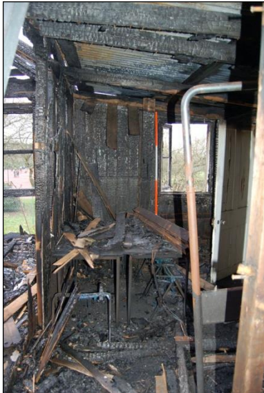
Plate 21: Room G5 looking west
