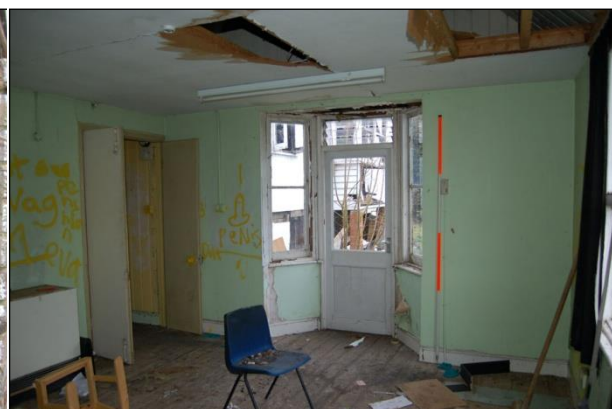
Plate 12: Room G1; west wall
