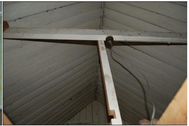
Plate 14: Room G1; roof
