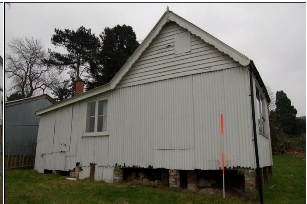
Plate 10: Building 2; north elevation
