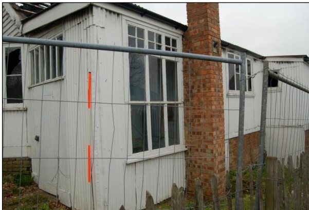
Plate 9: Building 1; north elevation
