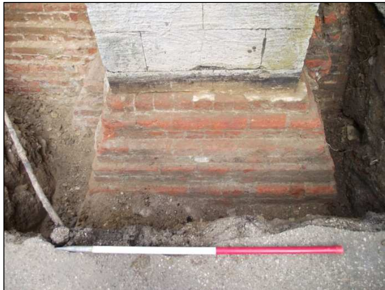
Plate 5: Church footings, looking NE ( scale 1m )
